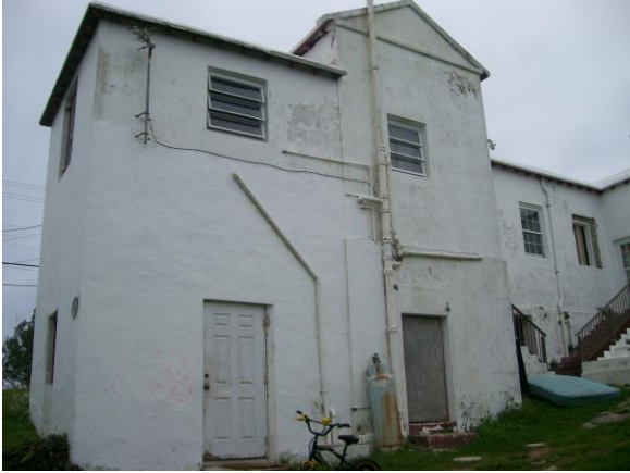
Lighthouse Apartment Complex
