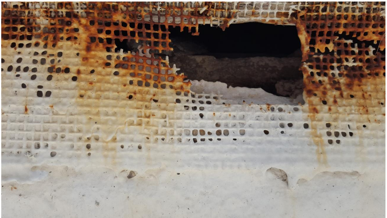
Main Roof Junction with Flat Roof
