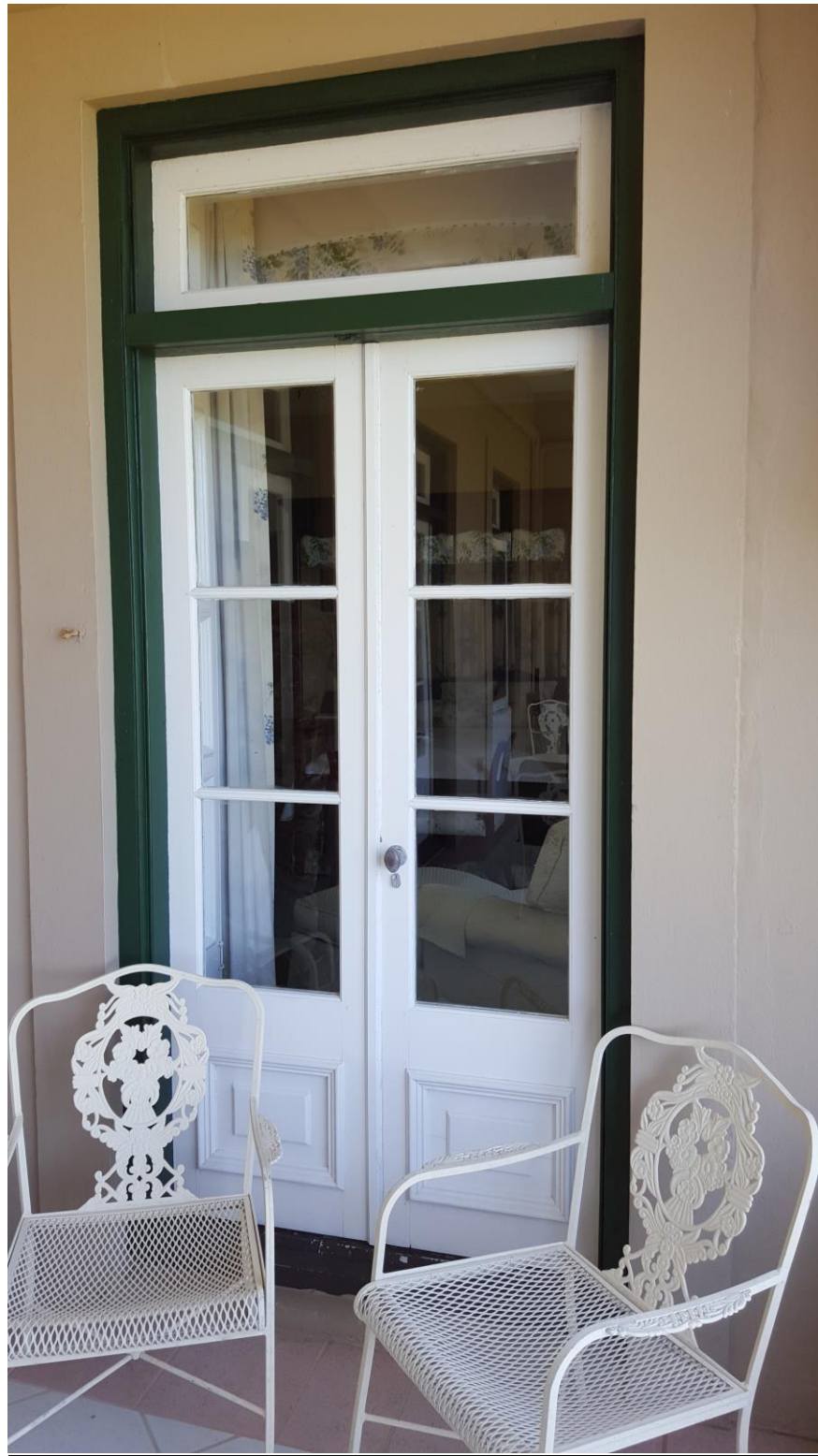
West Elevation Balcony French Doors
