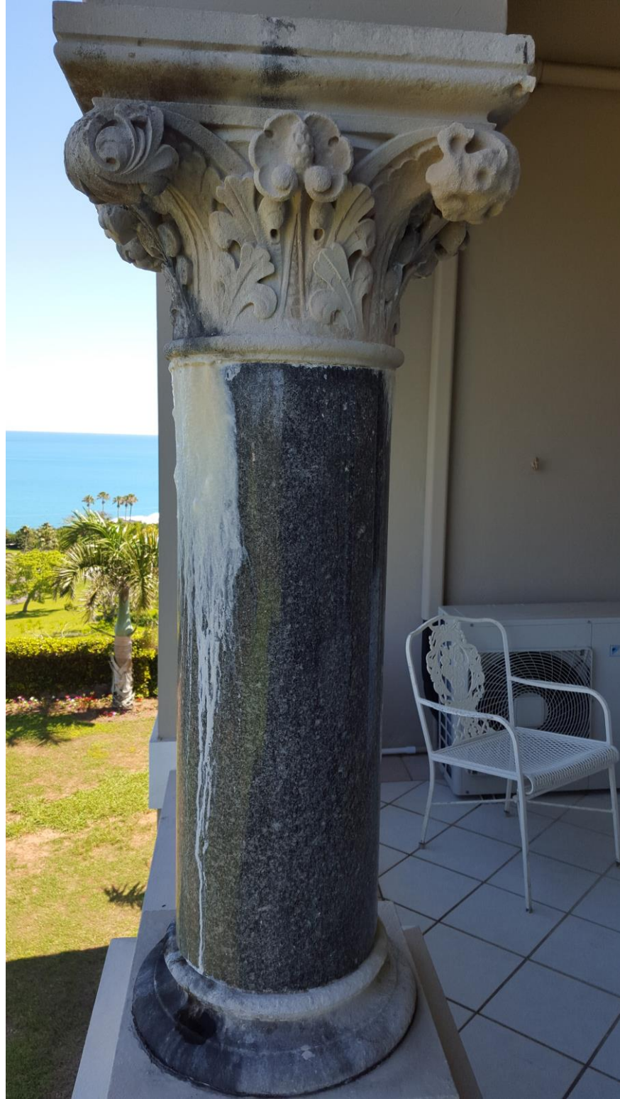
Calcification to Columns to West Elevation
