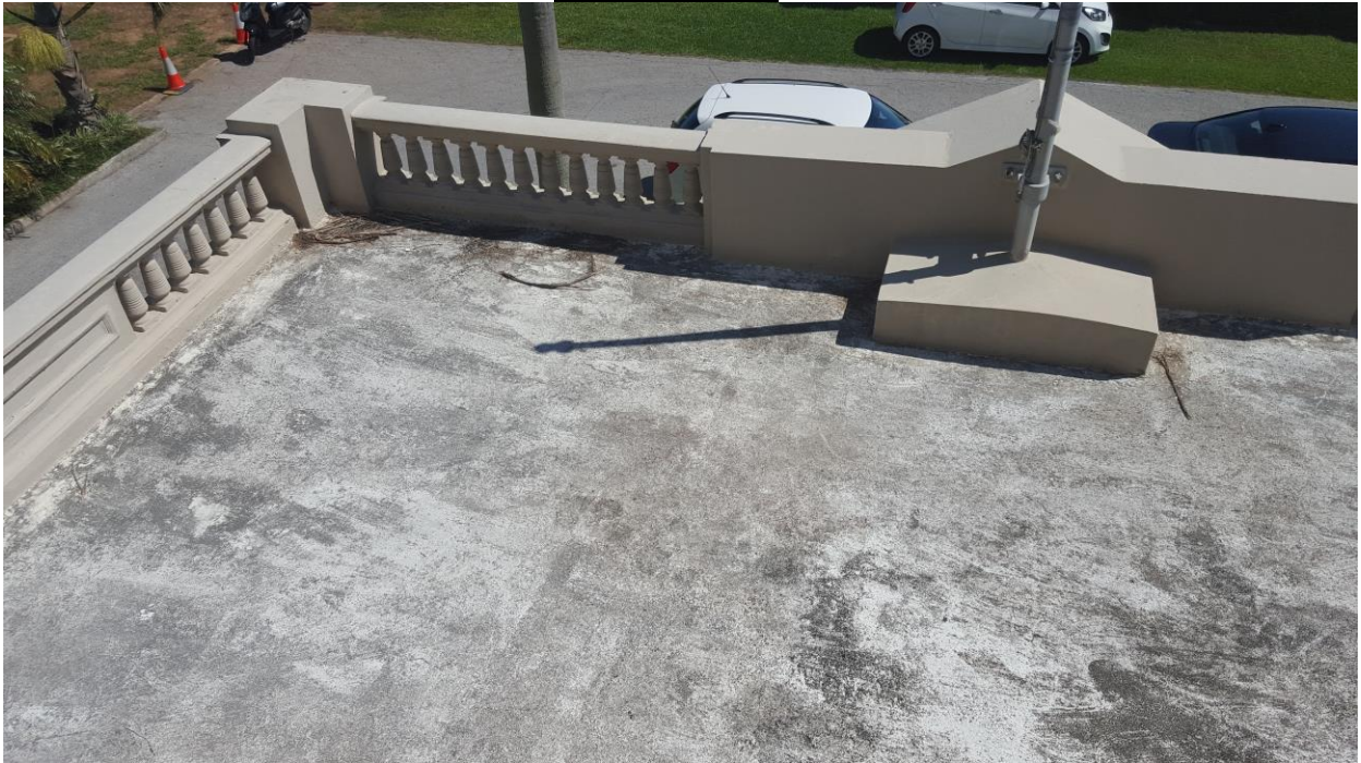
North Flat Roof above Main Entrance
