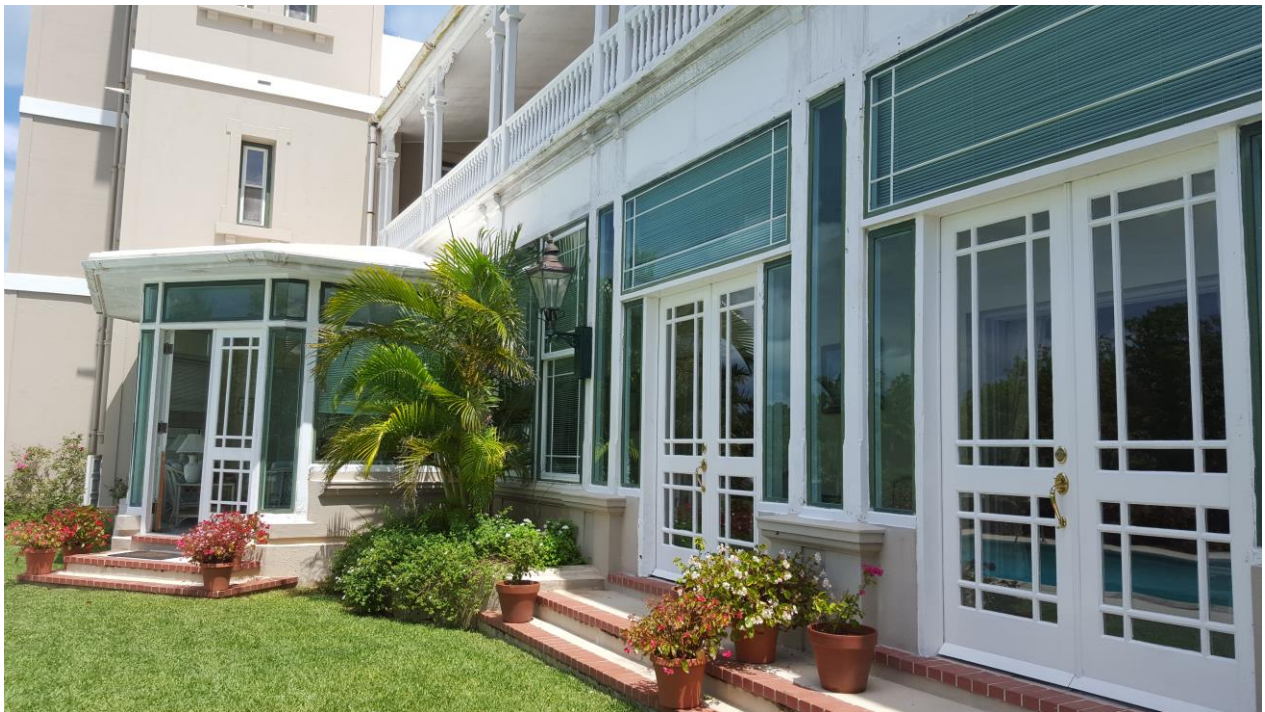
South/West Conservatory and Verandah
