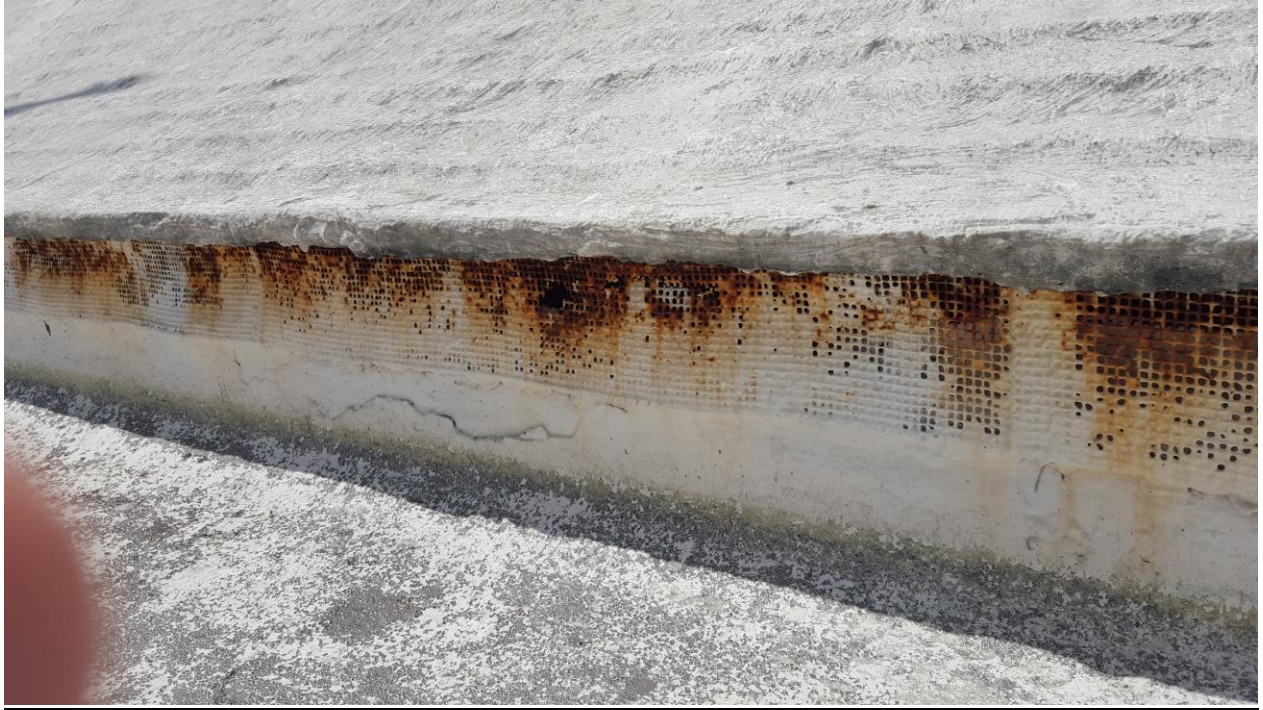
Main Roof Junction with Flat Roof
