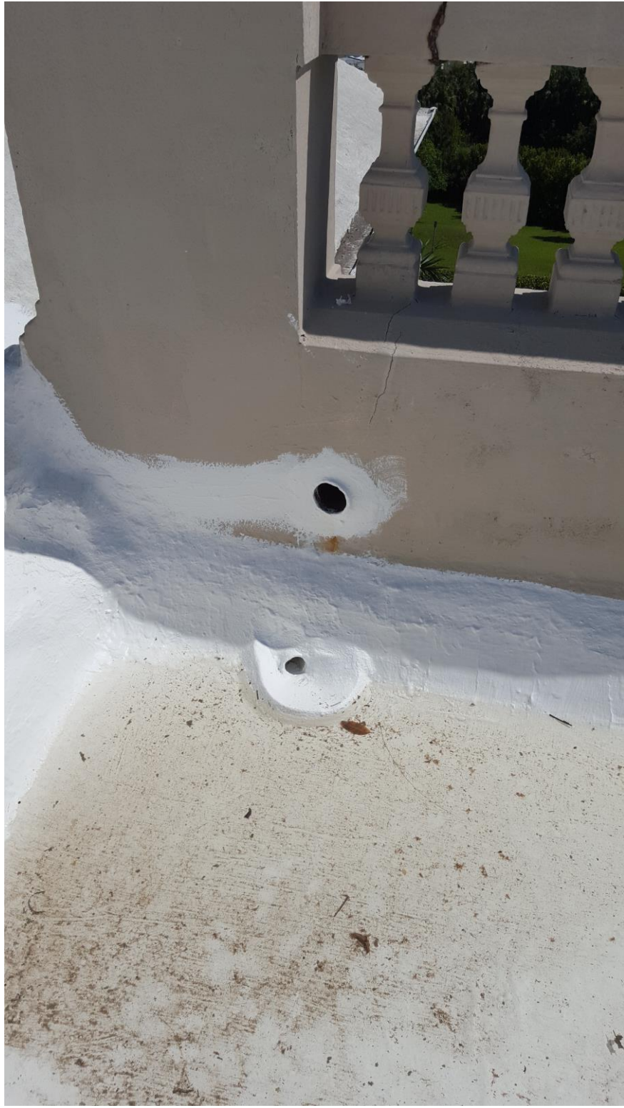
Flat Roof above Main Hallway
