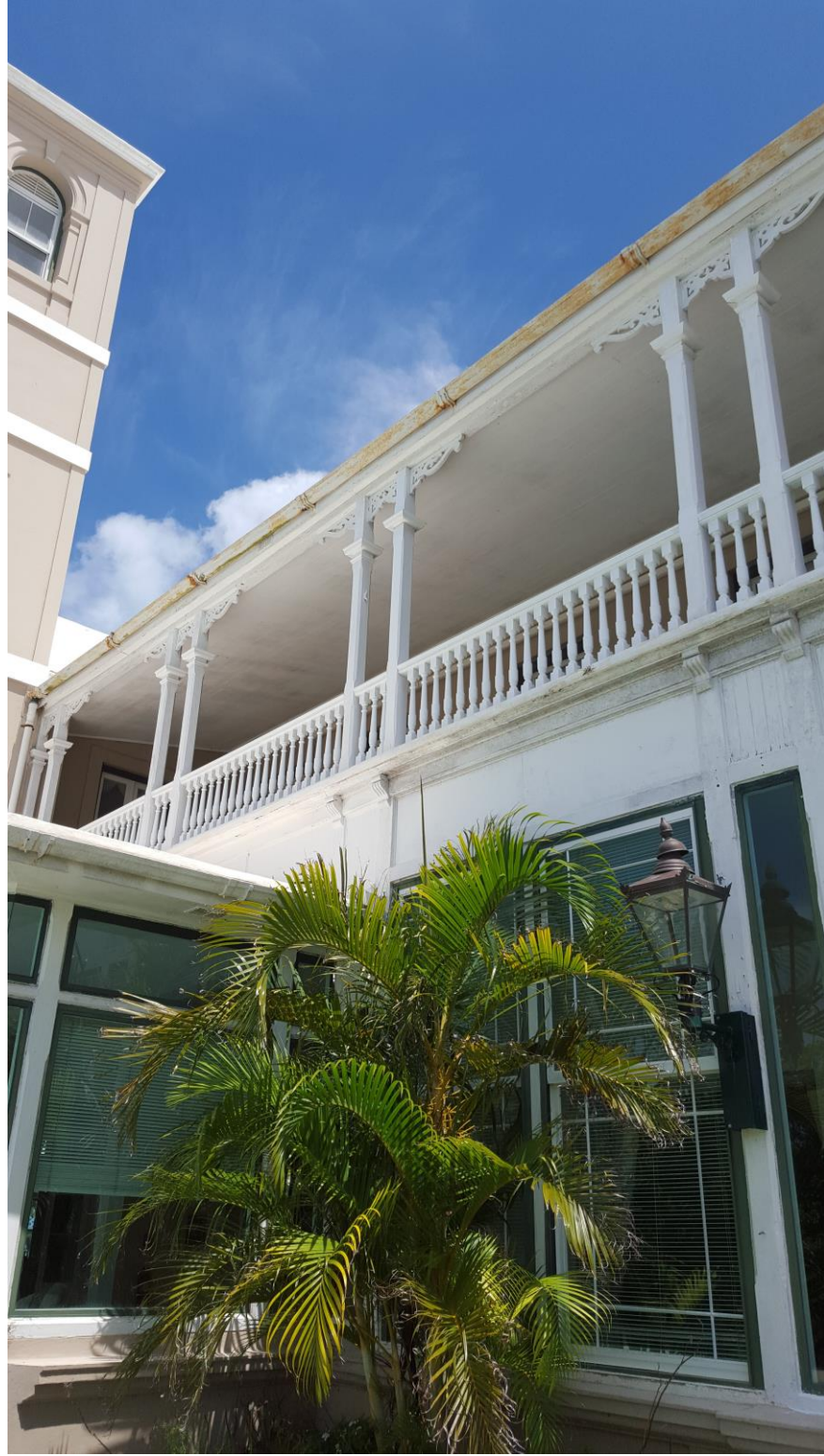
South Verandah and Conservatory
