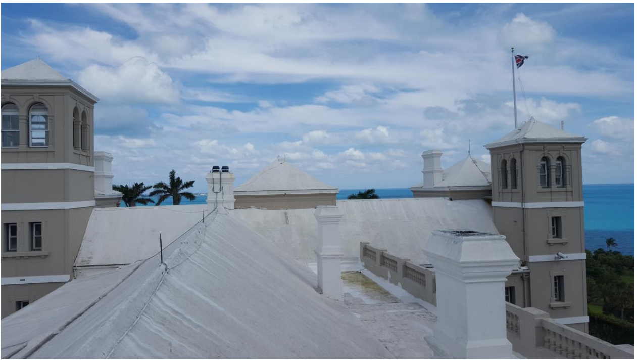
Main Roof West
