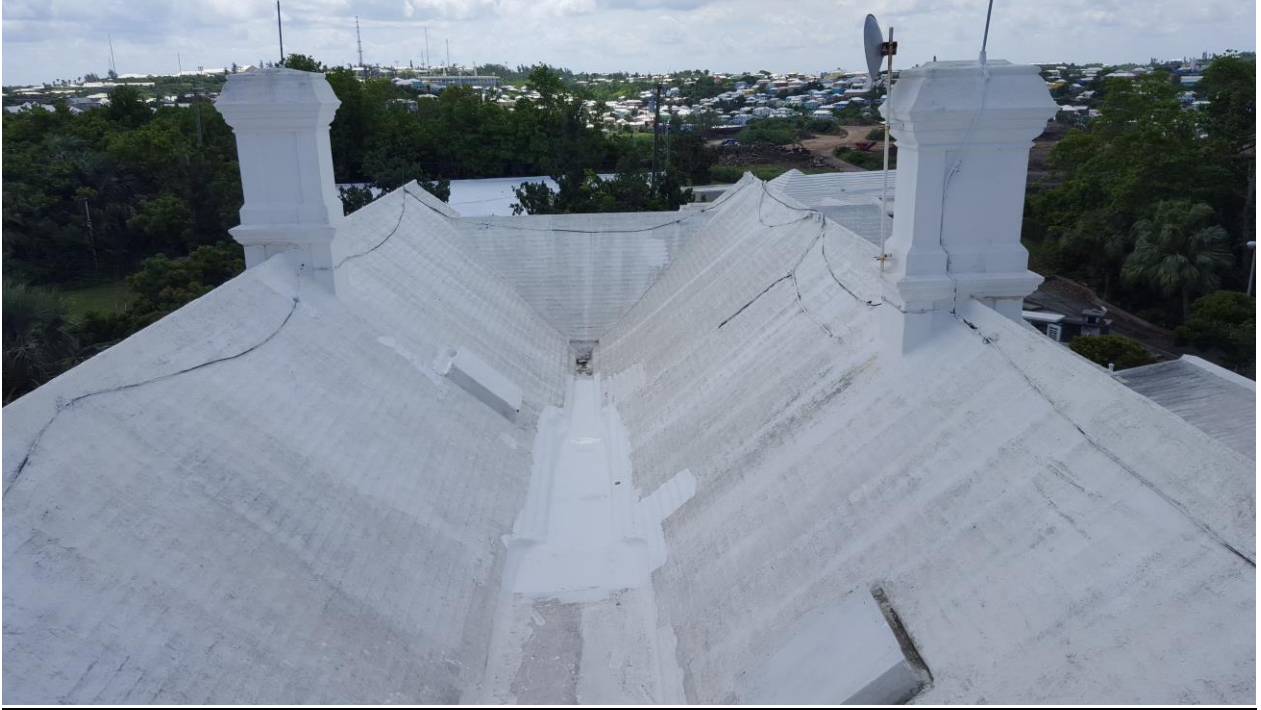
Main Roof East
