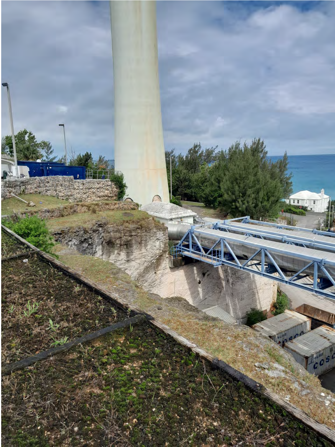
Photo 1 View of Monitoring Building
