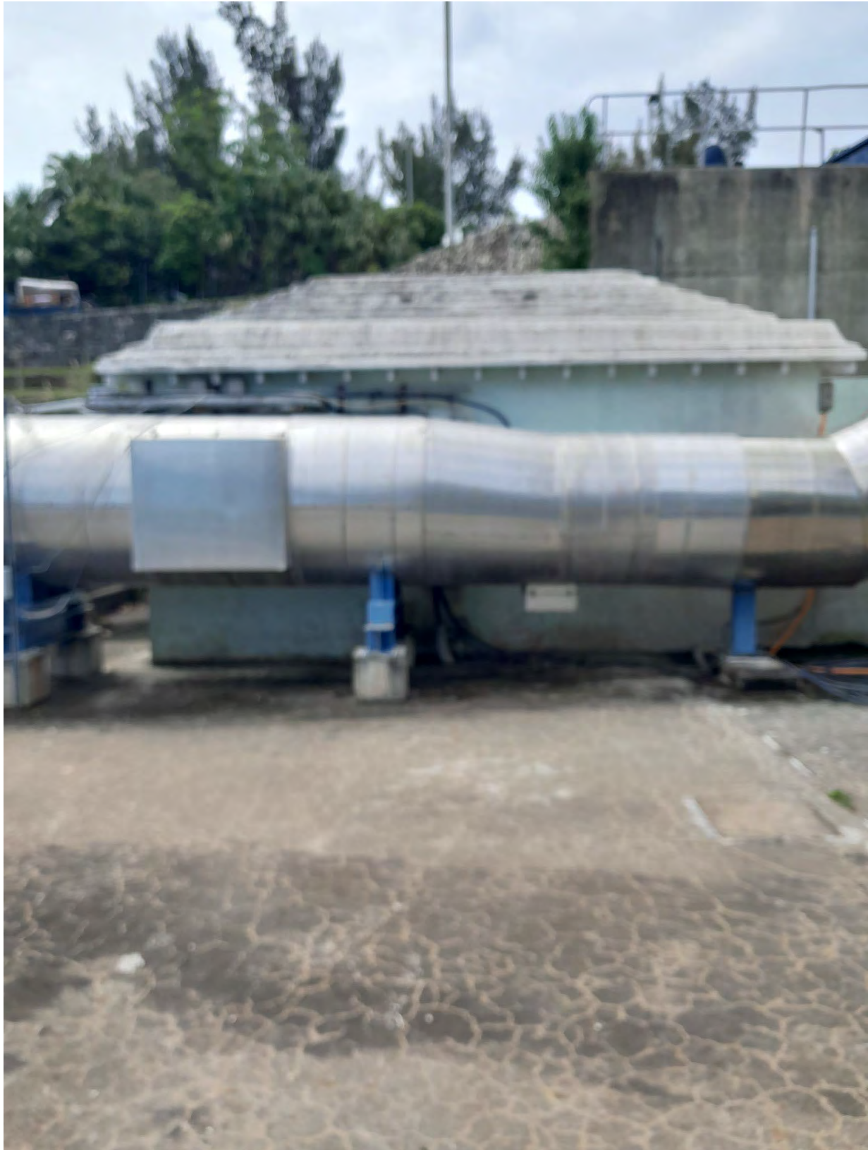
Photo 4 Exterior of Monitoring Building Looking Southward
