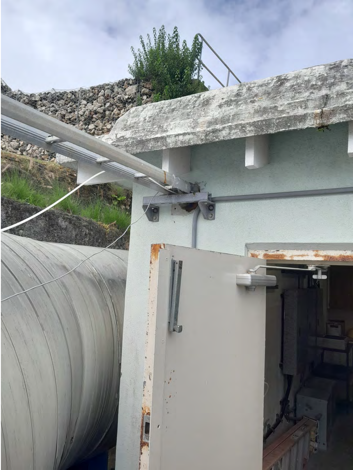
Photo 19 Existing Door Hardware
