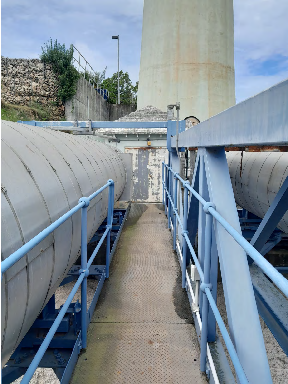
Photo 14 Existing Monitoring Building
