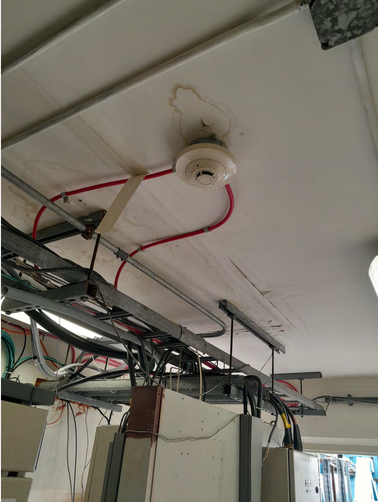
Photo 32 Repair Ceiling and Patch Water Leak
