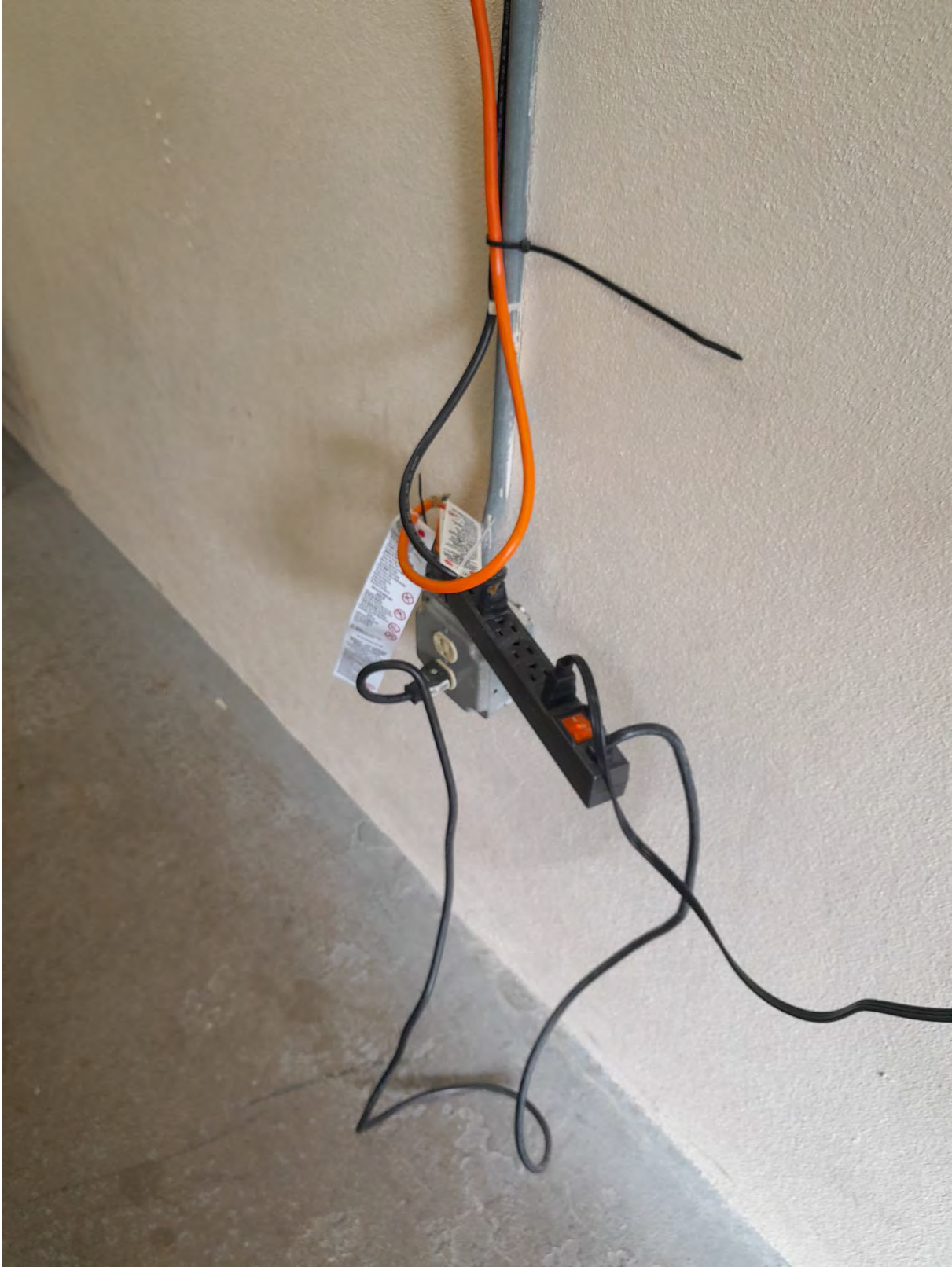
Photo 25 Power Bars to be Removed
