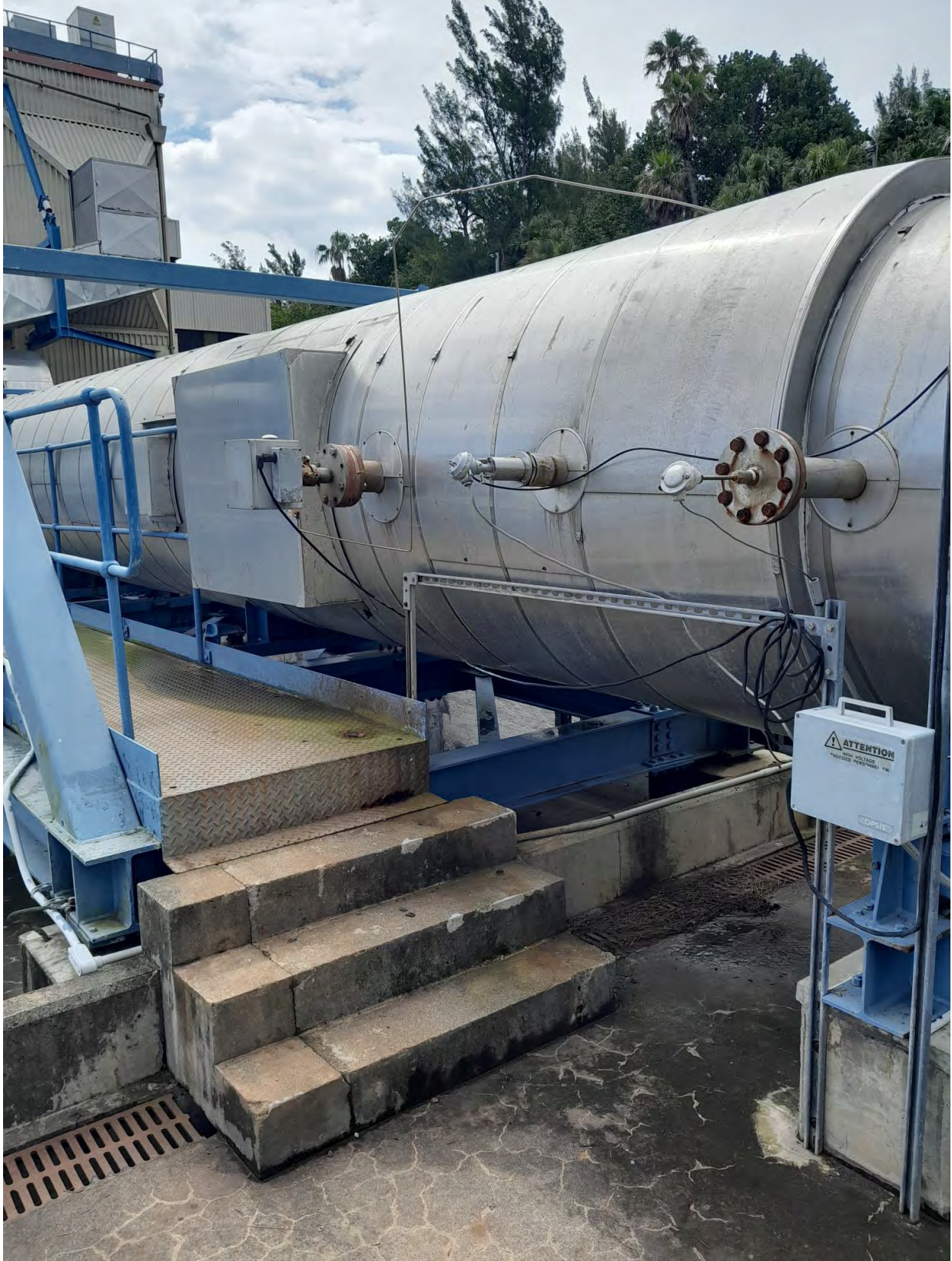
Photo 5 Typical CEMS Probe Locations
