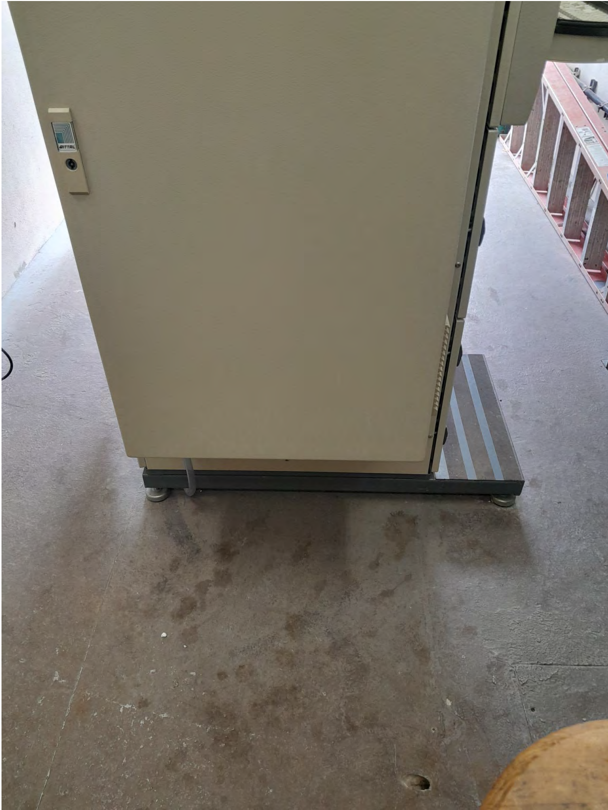
Photo 29 Floors to be Repaired and Painted
