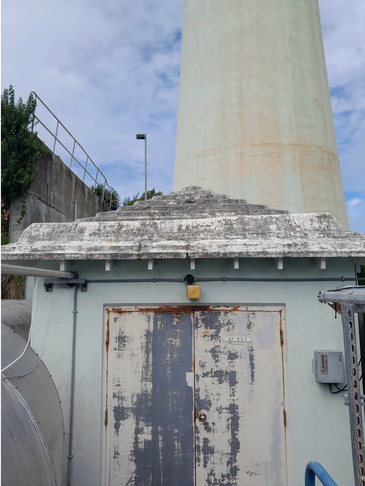
Photo 33 Exterior of Monitoring Building
