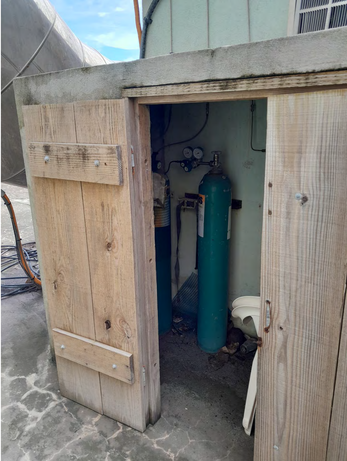
Photo 9 Existing Gas Bottle Shed
