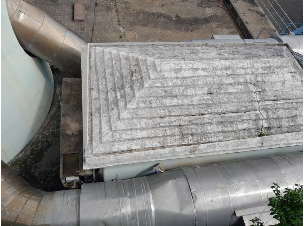
Photo 2 Monitoring Building Roof
