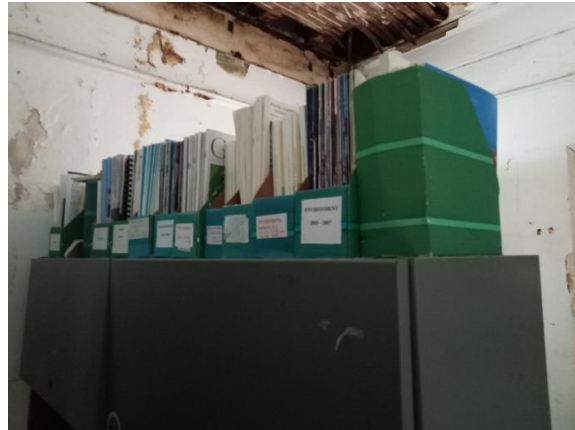
BGL- 26: Room 105, D7
