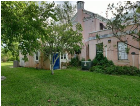
BGL- 35: Northwest Elevation
