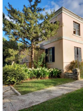
BGL- 34: Southwest Elevation
