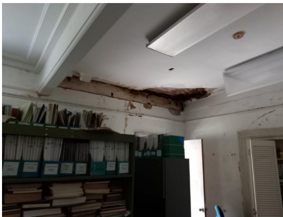
BGL- 31: Room 105, S5, D7
