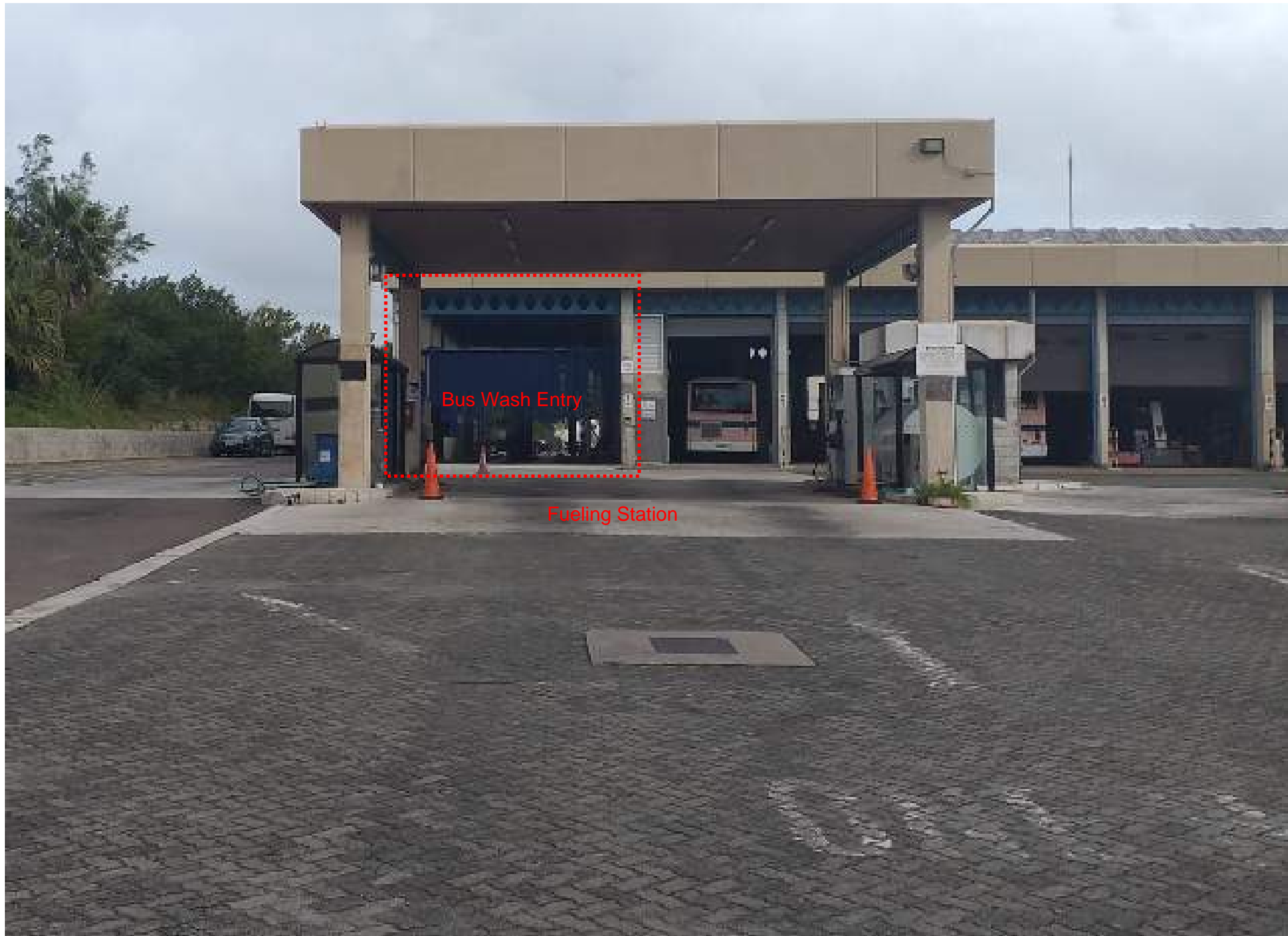
EXISTING BUS WASH ENTRANCE Fueling Station in foreground
