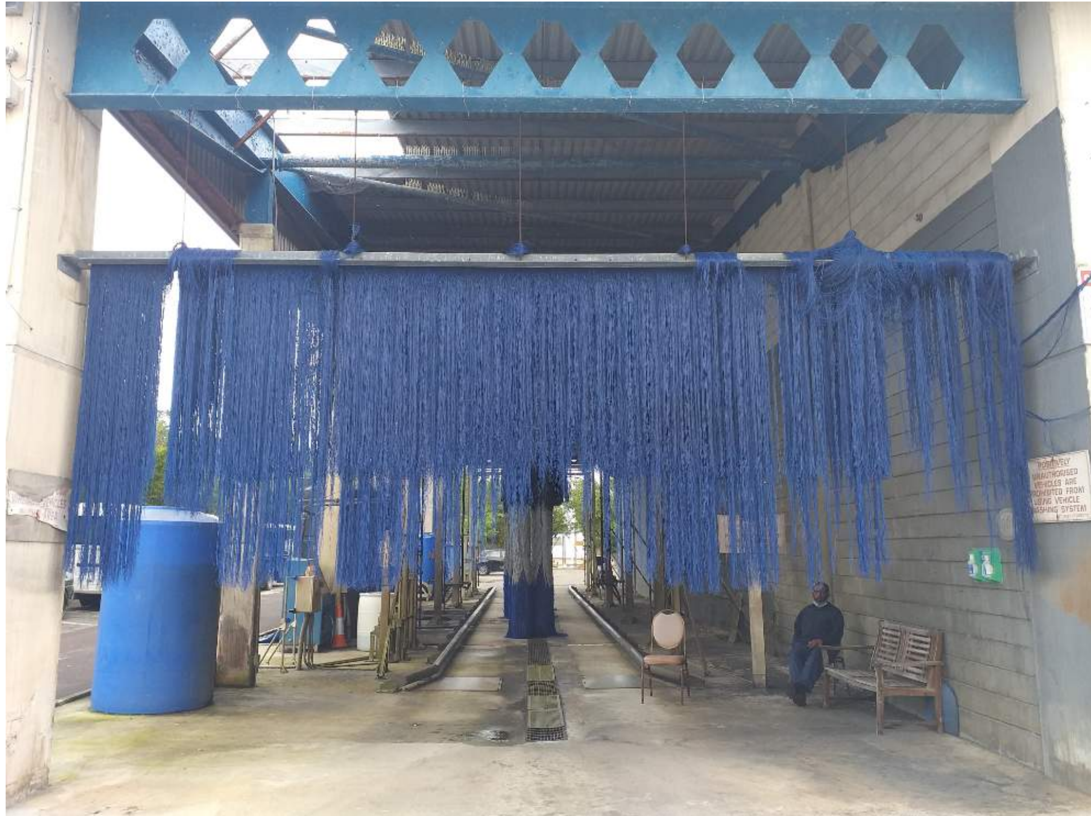
EXISTING BUS WASH ENTRANCE
