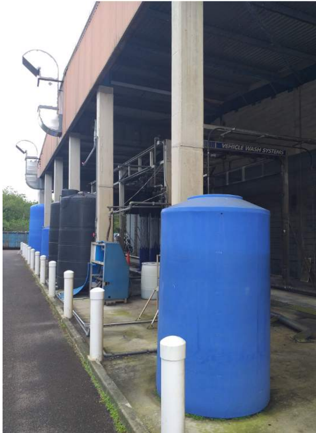
Bus Wash and water reclamation (View of the North Facade)
