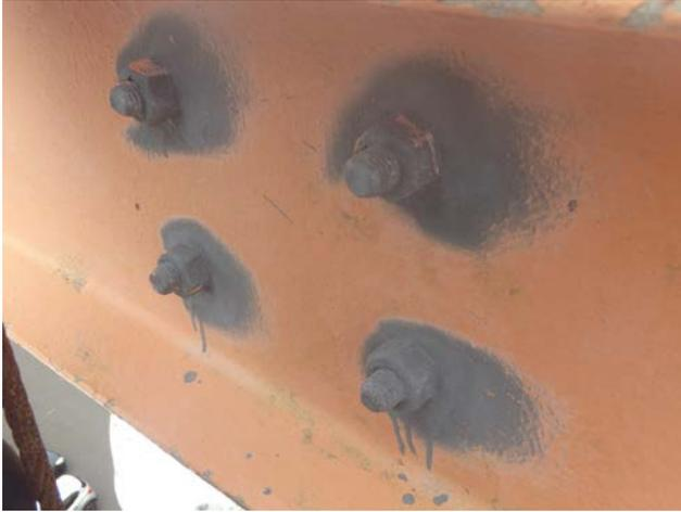
70' 6" torque arm bolt assemblies
