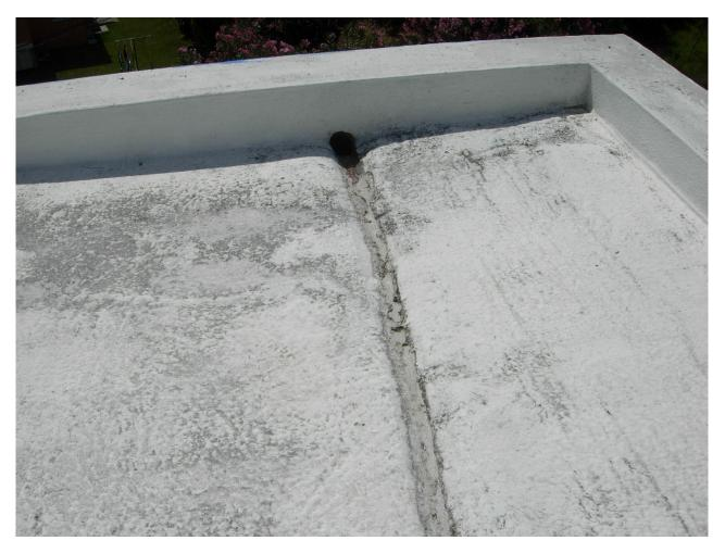
Typical Rainwater Drainage Channel and Outlet (1 of 4)
