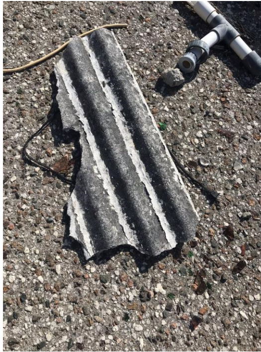
Sample KOBE 2B – Building A Roofing East – 20% Chrysotile
