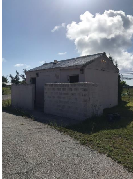
Sample KOBE 8B – Building B Roofing – 20% Chrysotile
