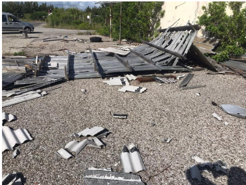
Roofing from Building A
