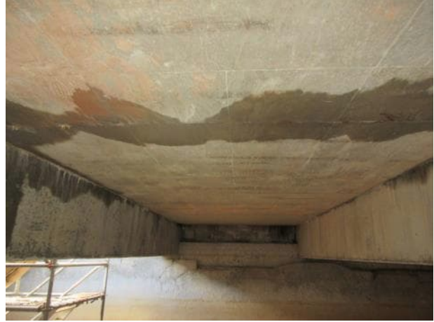
Photo 5.1.18. Underside of slabs between B2 and B3.
