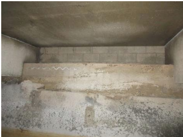
Photo 5.4.37 South bearing area between B18 and B19.
