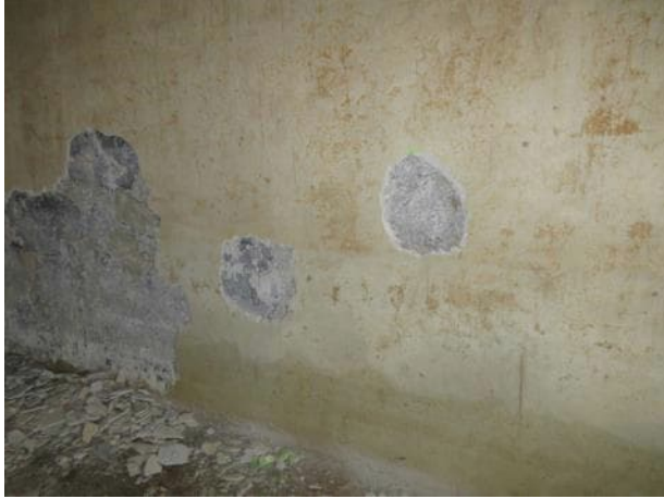
Photo 5.5.3 North wall section 3.
