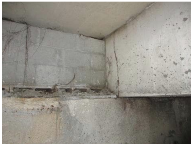
Photo 5.2.32. B10 north bearing.
