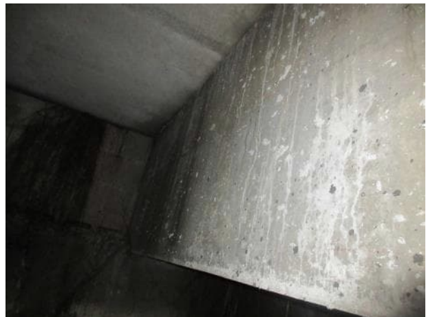
Photo 5.3.4. B11 looking north - west side.
