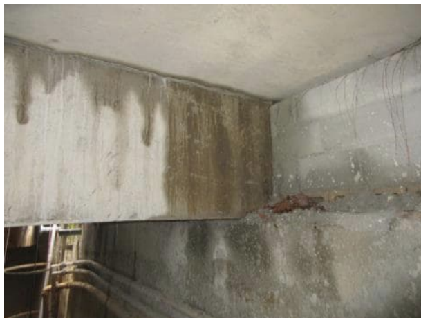
Photo 5.2.34. B9 north bearing.
