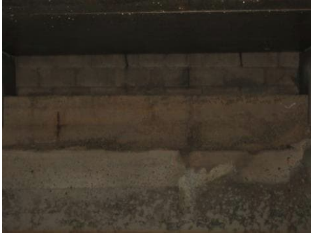
Photo 5.4.29 South bearing area between B19 and B20.
