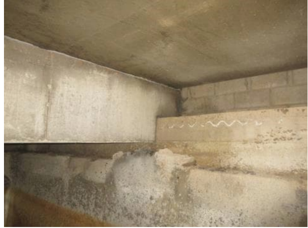
Photo 5.4.36 South bearing B19.
