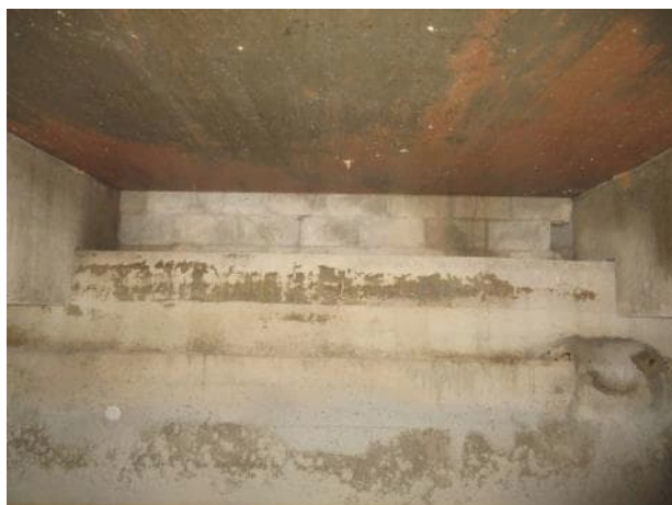
Photo 5.3.49. South bearing area between B14 and B15.
