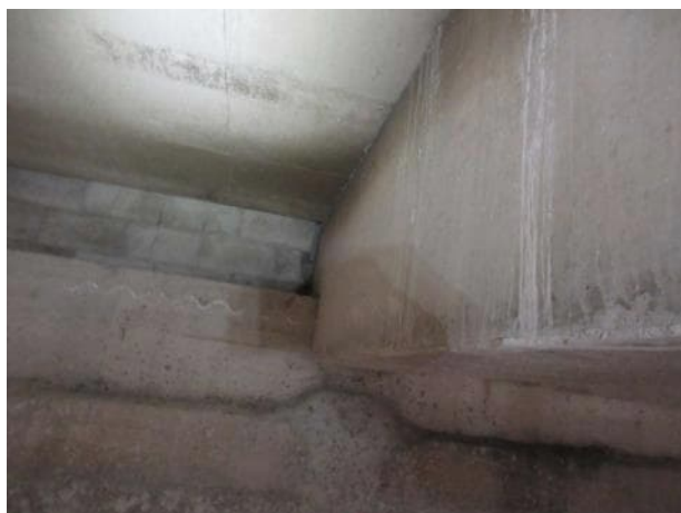
Photo 5.2.17. B8 south bearing.
