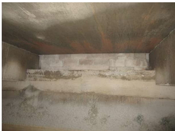
Photo 5.3.37. South bearing area between B12 and B13.
