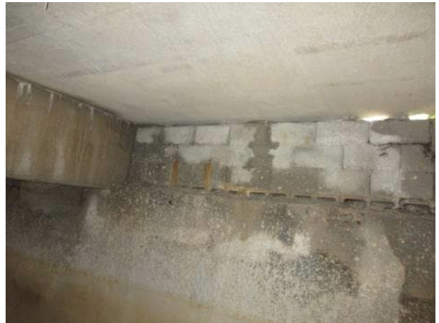
Photo 5.2.48. North bearing area between B5 and B6.
