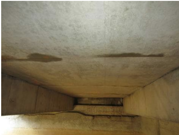
Photo 5.1.9. Slab between B1 and B2.
