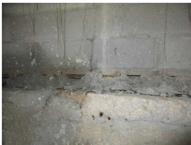
Photo 5.2.35. North bearing area between B9 and B10.
