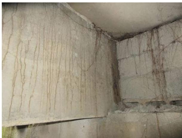
Photo 5.3.22. B14 north bearing east side.
