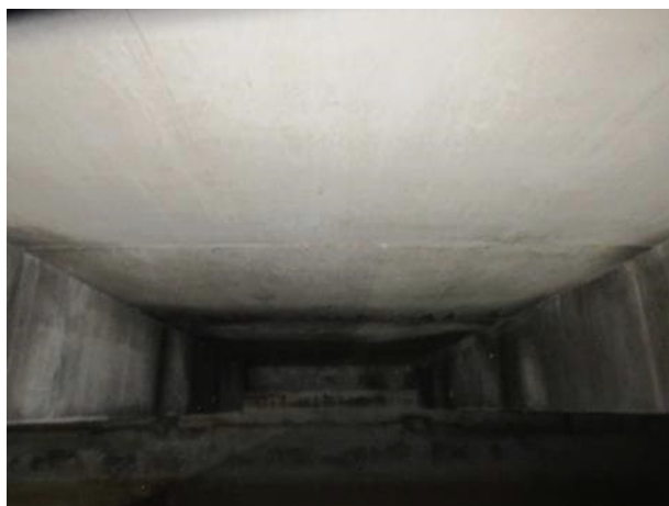
Photo 5.3.28. Slabs between B14 and B15.
