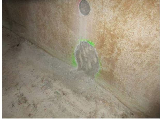
Photo 5.5.16 North wall Section 4.
