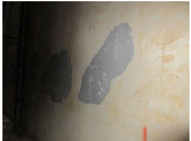
Photo 5.5.6 North wall section 2.
