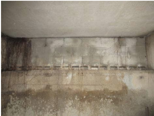
Photo 5.3.9. North bearing area between B12 and B13.
