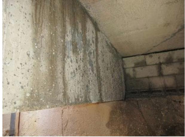
Photo 5.1.36. Beam B5 looking north.
