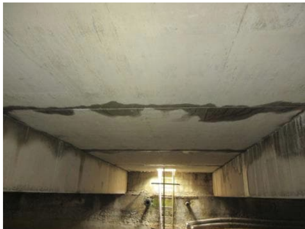
Photo 5.2.13. Underside of slab between B7 and B8.
