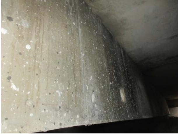
Photo 5.3.5. B11 looking west.
