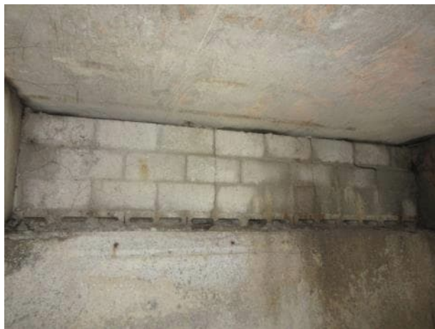
Photo 5.1.13. North bearing area between B2 and B3.
