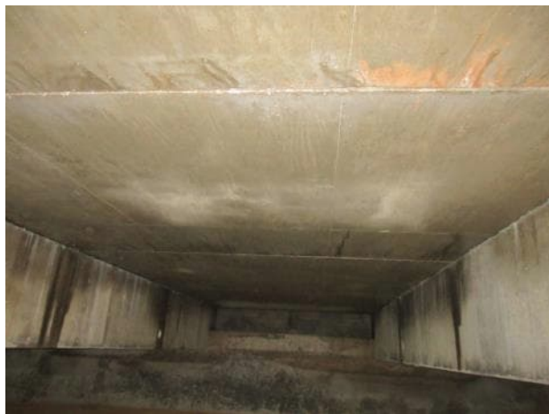
Photo 5.4.13 Underside of slabs between B17 and B18.
