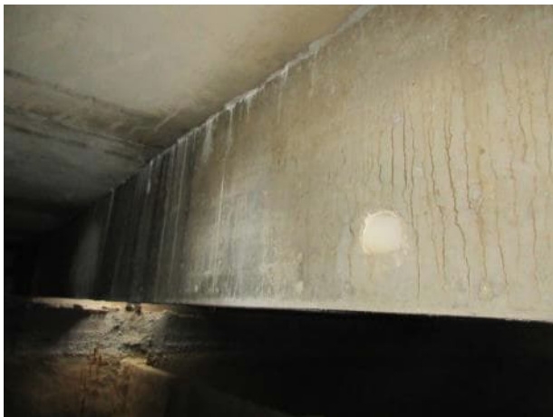
Photo 5.3.3. Beam B11 looking south.
