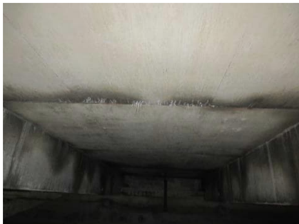
Photo 5.3.19. Slabs between B13 and B14.
