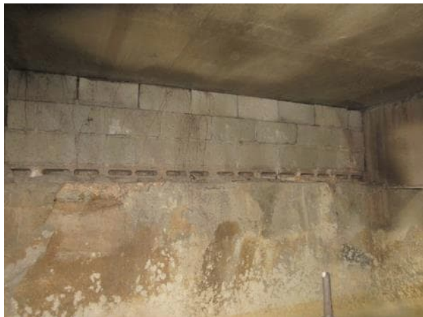
Photo 5.4.5 North bearing area between B16 and B17.
