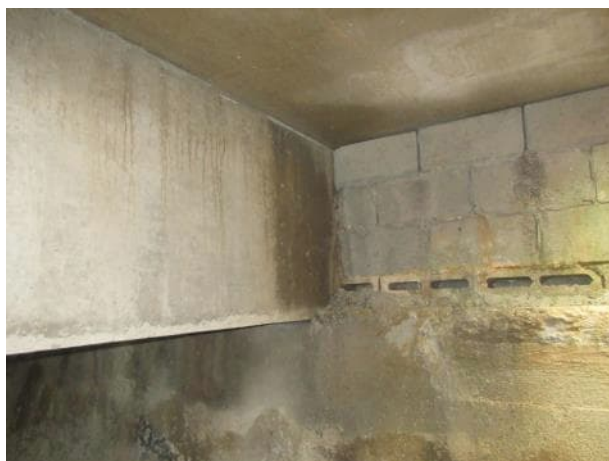
Photo 5.4.10 North bearing B17.
