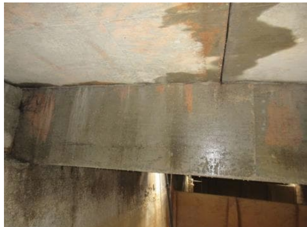
Photo 5.1.16. Beam B3 north end.
