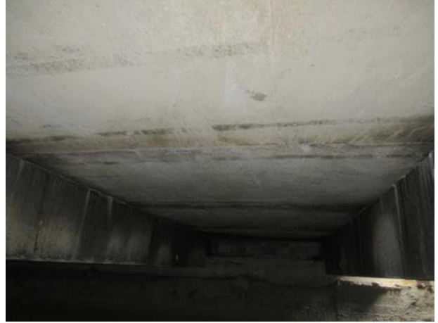
Photo 5.3.6. Slabs between B11 and B12.
