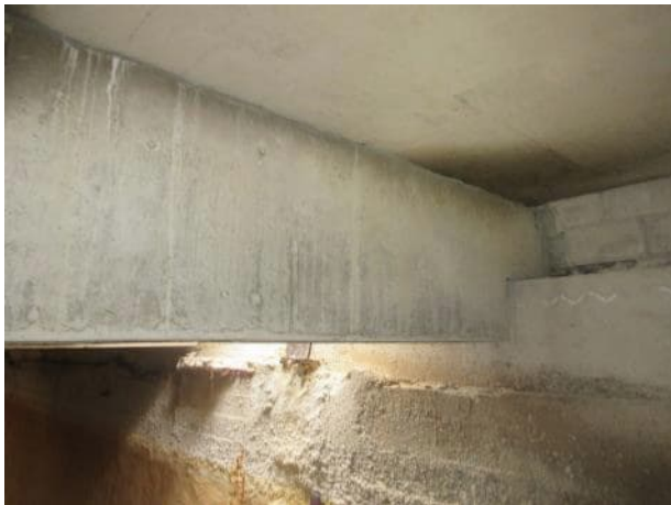
Photo 5.2.27. B10 south bearing.
