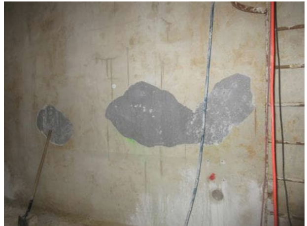
Photo 5.5.8 North wall section 2.
