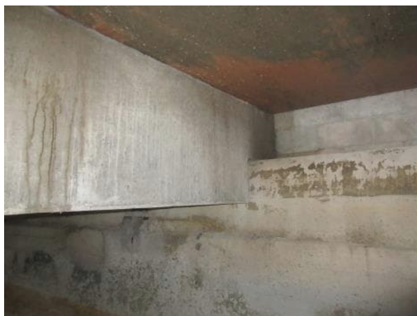
Photo 5.3.50. South bearing B15.
