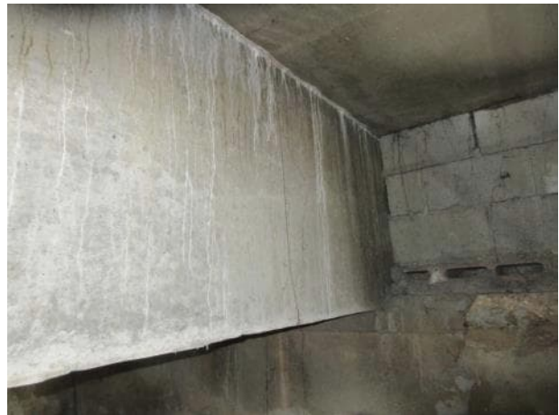
Photo 5.4.4 North bearing B16.
