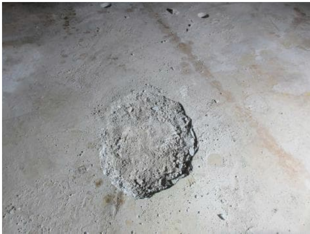
Photo 5.5.17 Hollow floor coating in Section 4 south side.
