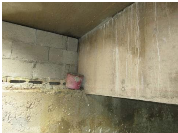
Photo 5.4.14 North bearing B18.
