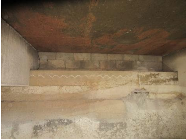
Photo 5.4.47 South bearing area between B15 and B16.
