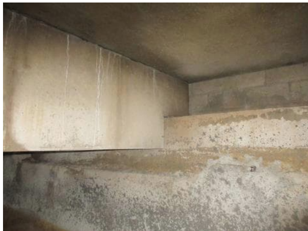
Photo 5.4.41 South bearing B18.
