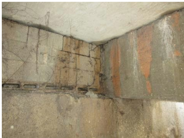
Photo 5.1.25. Beam B4 north bearing.
