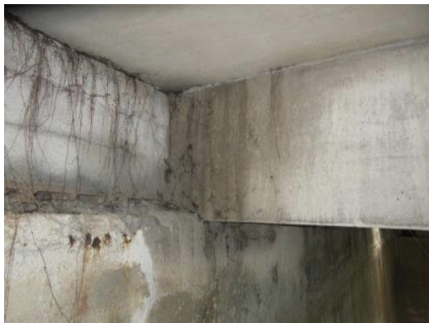
Photo 5.3.26. B15 north bearing.
