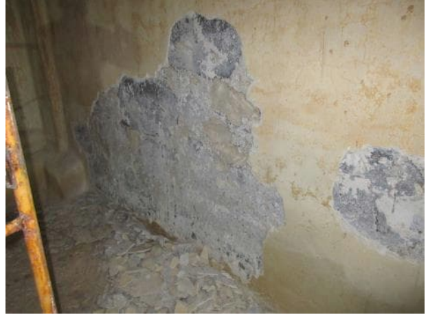
Photo 5.5.4 North wall section 3.
