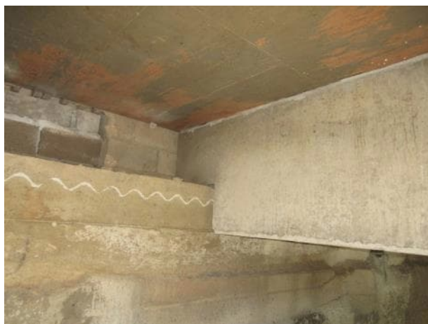
Photo 5.4.46 South bearing B16.
