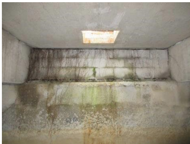
Photo 5.3.16. North bearing area between B13 and B14.
