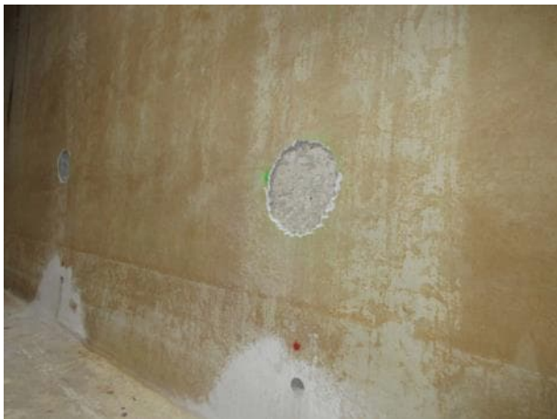
Photo 5.5.13 North wall section 1.
