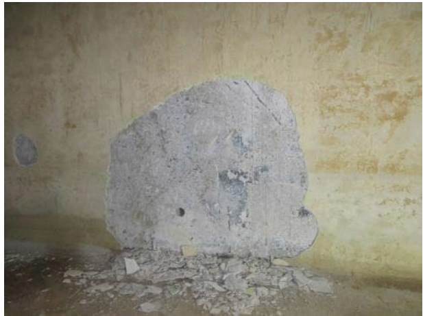
Photo 5.5.2 North wall section 3.
