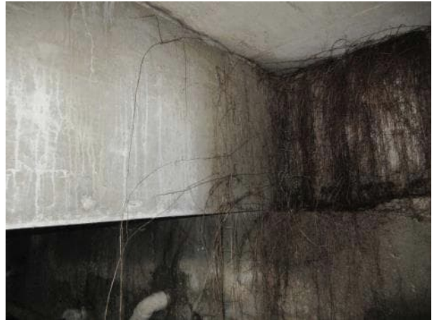
Photo 5.3.2. North bearing B11.
