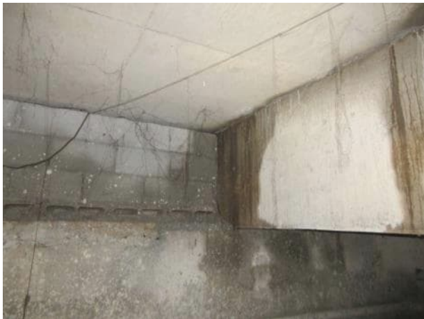
Photo 5.2.39. B9 north bearing.
