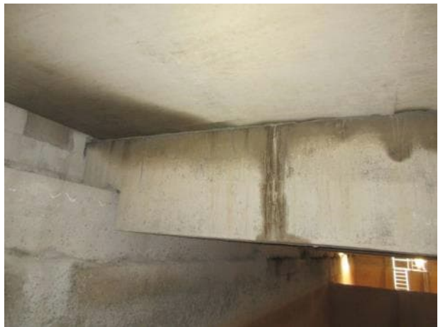
Photo 5.2.24. B9 south bearing.
