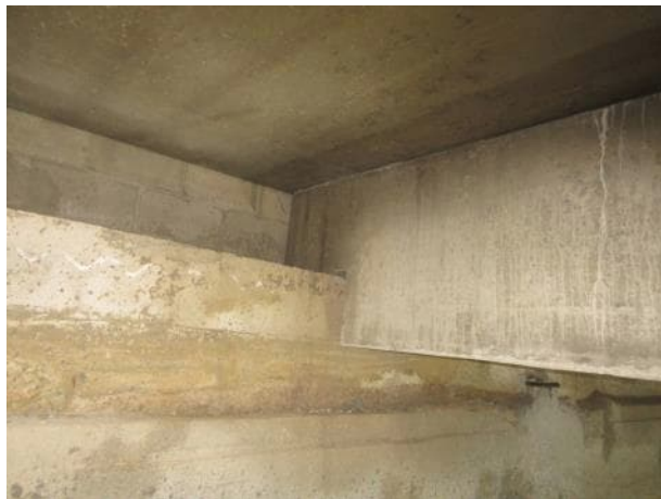
Photo 5.4.42 South bearing B17.
