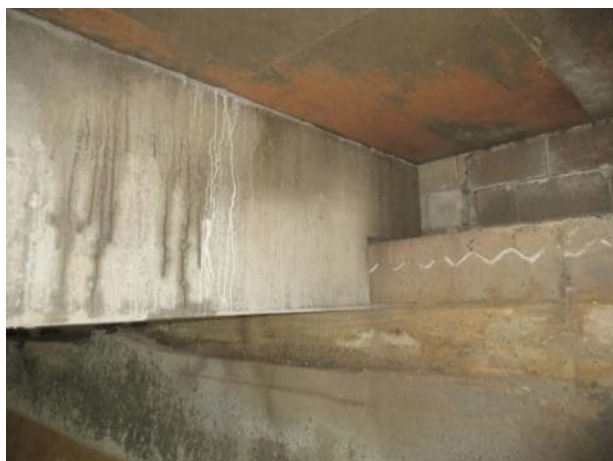
Photo 5.4.45 South bearing B17.
