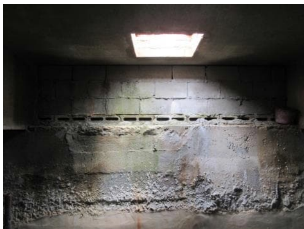
Photo 5.4.9 North bearing area between B17 and B18.
