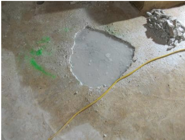
Photo 5.5.1 Hollow section in Section 3 Floor (eastern end).
