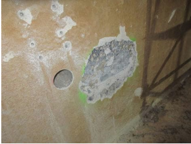
Photo 5.5.15 North wall Section 4.
