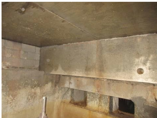
Photo 5.4.27 North bearing B20.
