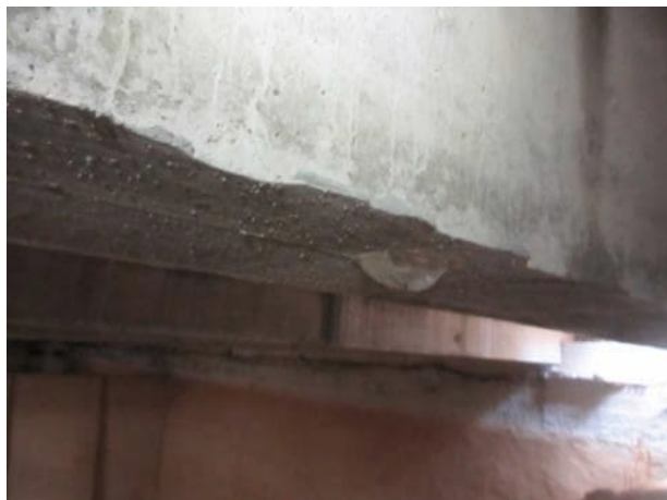
Photo 5.2.33. B10 plastic on the underside of the beam likely from the initial installation. No structural issue.
