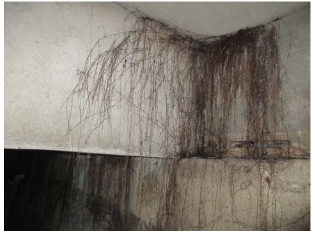
Photo 5.3.10. B12 north bearing.
