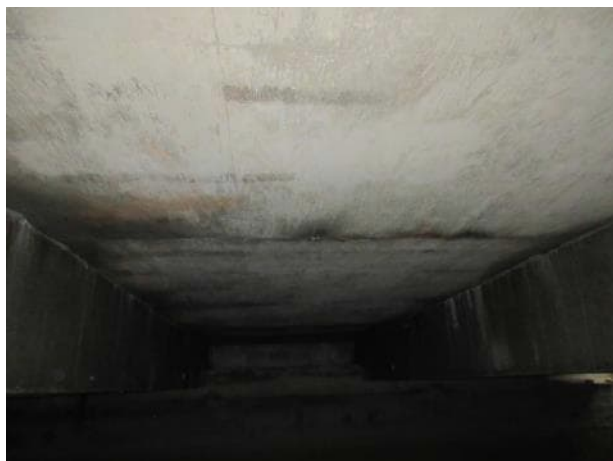
Photo 5.3.15. Slabs between B12 and B13.
