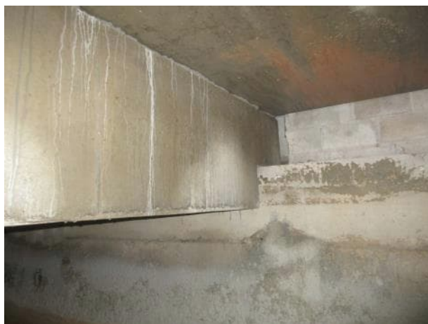
Photo 5.3.38. B13 south bearing.
