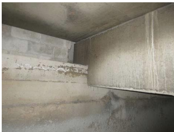
Photo 5.3.40. South bearing B13.
