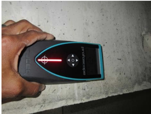
Photo 5.1.11. Rebar scan of B1.
