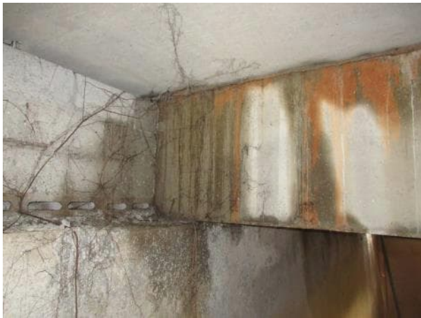
Photo 5.1.7. B2 north bearing.
