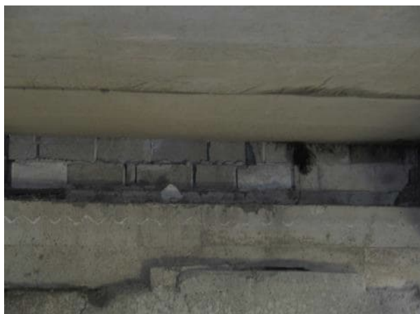
Photo 5.1.33. South bearing area between B4 and B5.
