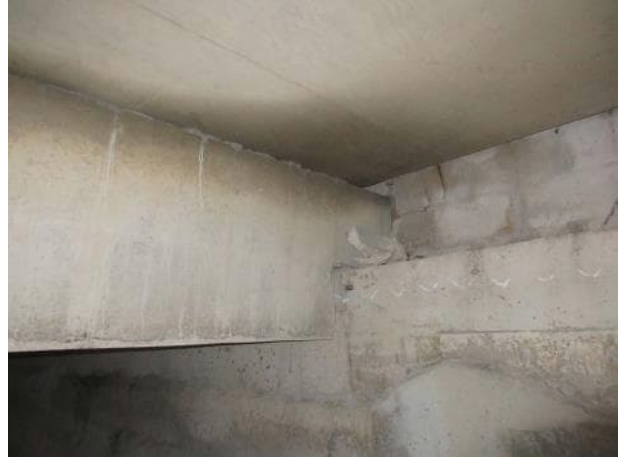
Photo 5.2.8. B7 south bearing.
