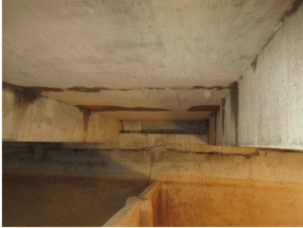
Photo 5.1.35. Underside of slab between B5 and B6.
