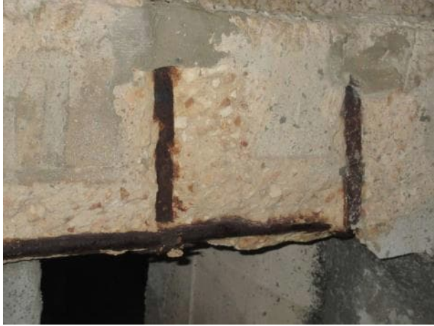
Photo 5.4.35 Corroded stirrups.
