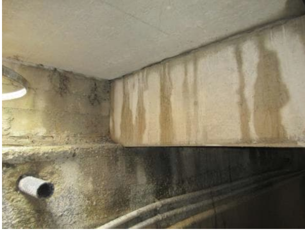
Photo 5.2.43. B8 north bearing.
