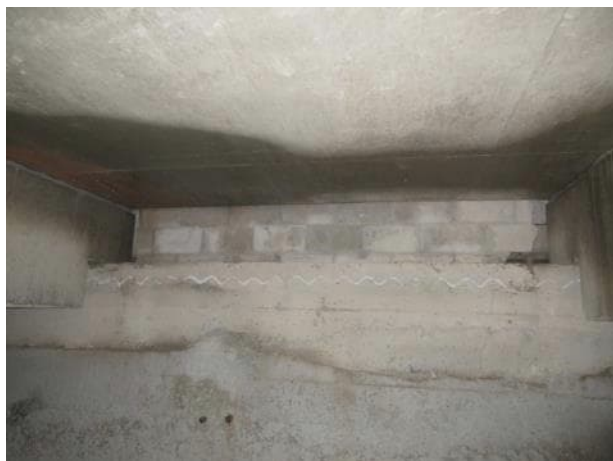
Photo 5.3.33. South bearing area between B11 and B12.
