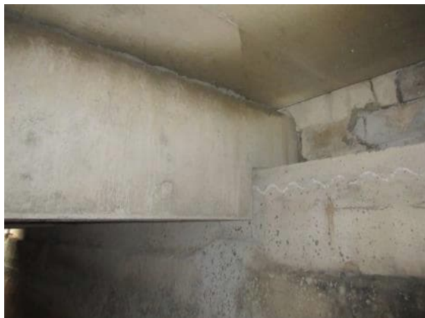
Photo 5.2.15. B8 south bearing.
