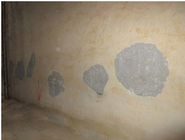
Photo 5.5.5 North wall section 2.
