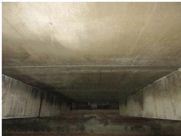
Photo 5.4.8 Underside of slabs between B16 and B17.
