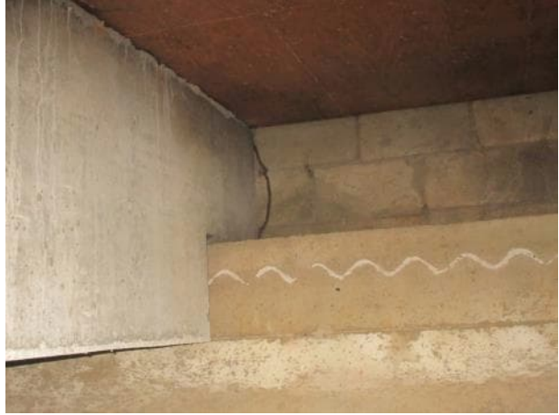
Photo 5.4.48 South bearing B16.
