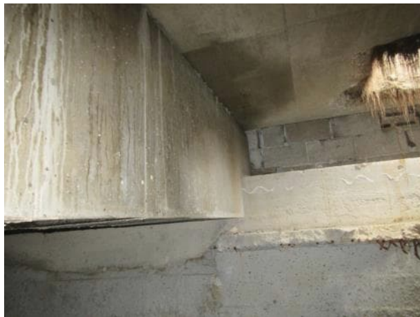
Photo 5.3.30. Beam B11 south bearing.
