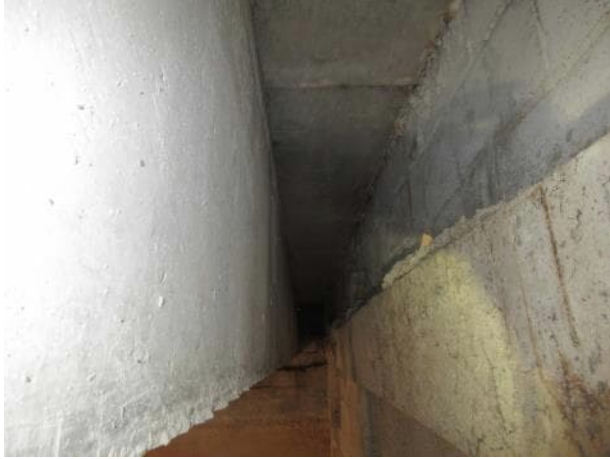
Photo 5.1.5. B1 looking toward south bearing.
