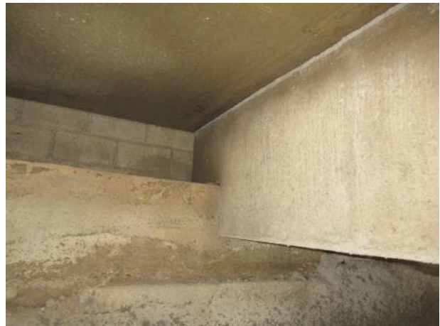
Photo 5.4.38 South bearing B18.
