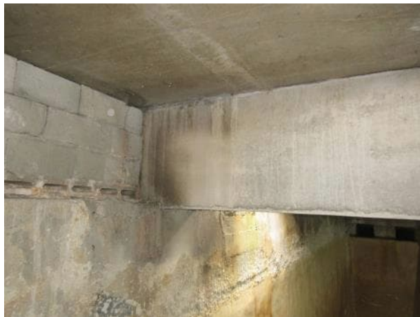
Photo 5.4.6 North bearing B17.
