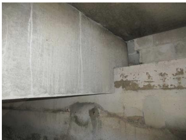
Photo 5.3.46. South bearing B14.
