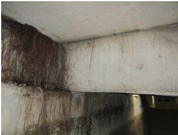
Photo 5.3.7. North bearing B12.
