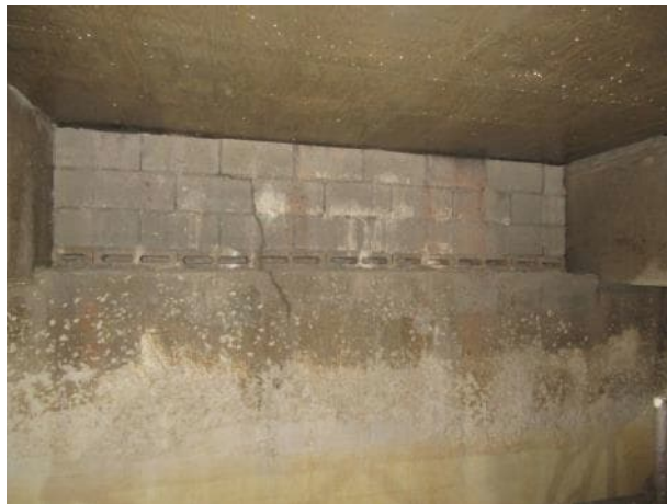
Photo 5.4.24 North bearing between B19 and B20.
