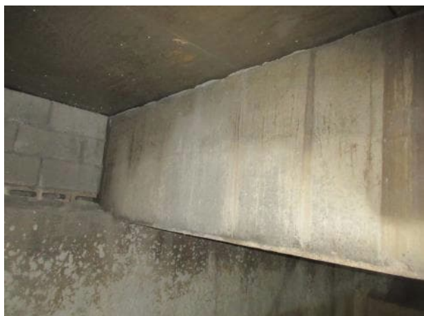
Photo 5.4.22 North bearing B19.
