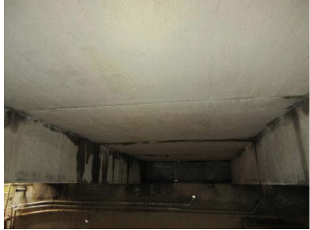
Photo 5.2.26. Underside of slab between B9 and B10.
