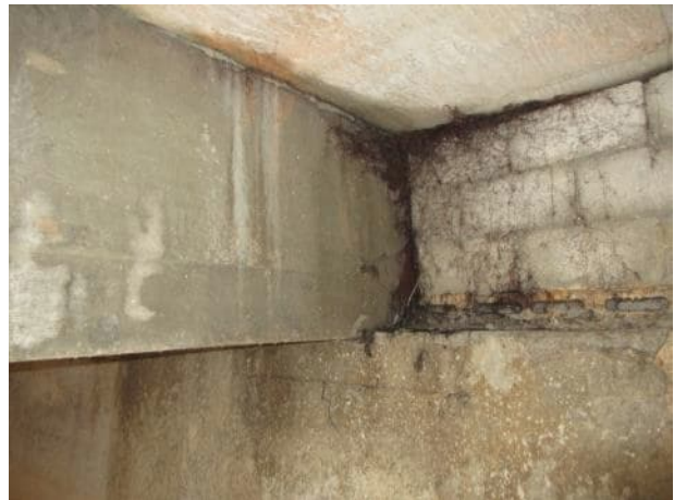
Photo 5.1.20. North bearing of B3. Roots visible.
