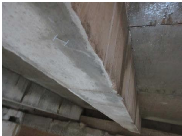
Photo 5.4.15 Underside of Beam B18.
