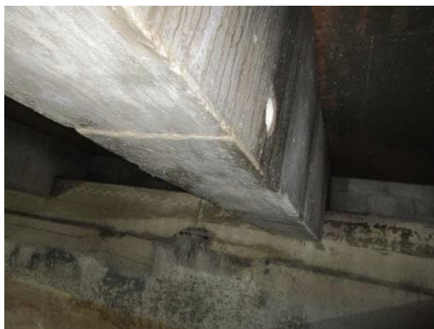
Photo 5.3.52. Underside of B15.
