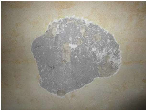
Photo 5.5.7 North wall section 2.
