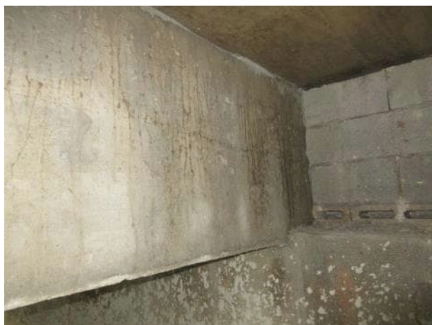
Photo 5.4.25 North bearing B19.
