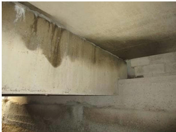
Photo 5.2.23. B9 south bearing.
