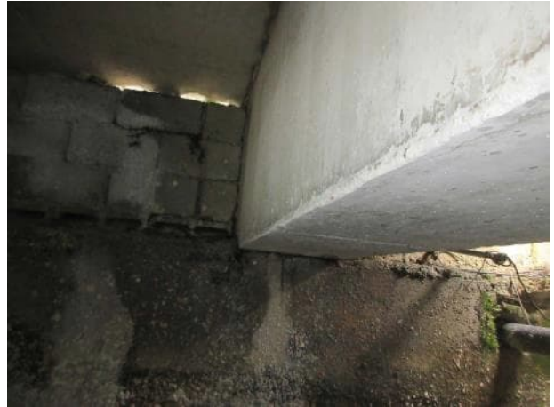
Photo 5.2.46. B6 north bearing.
