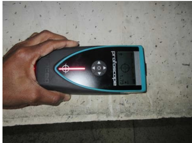
Photo 5.1.12. Rebar scan of B1.
