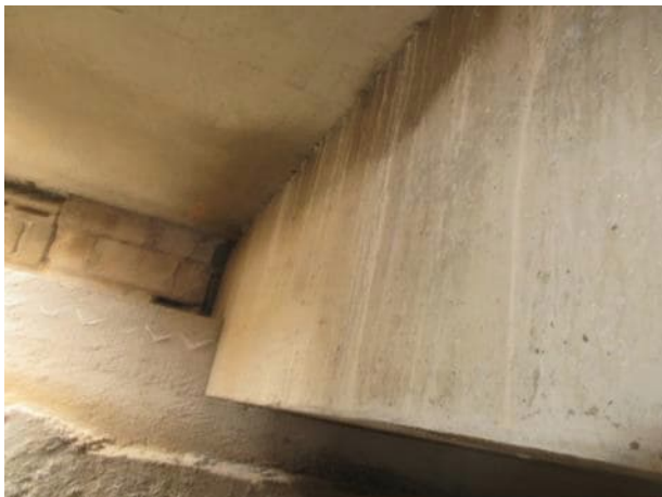
Photo 5.2.29. B10 south bearing.
