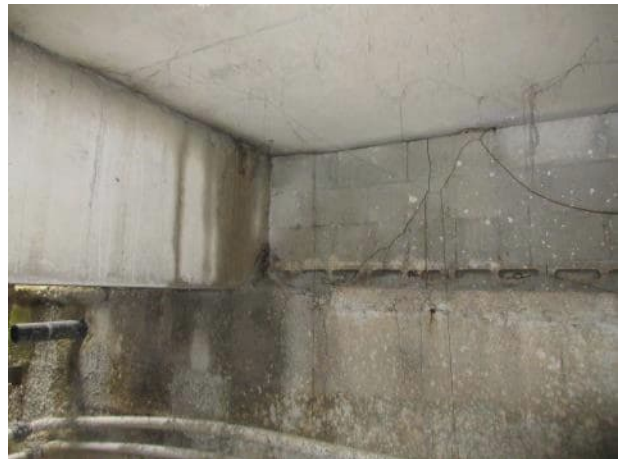
Photo 5.2.40. B8 north bearing.
