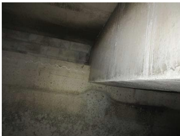
Photo 5.2.18. B8 south bearing.
