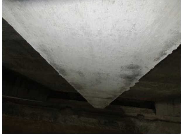
Photo 5.4.2. Underside of B16.
