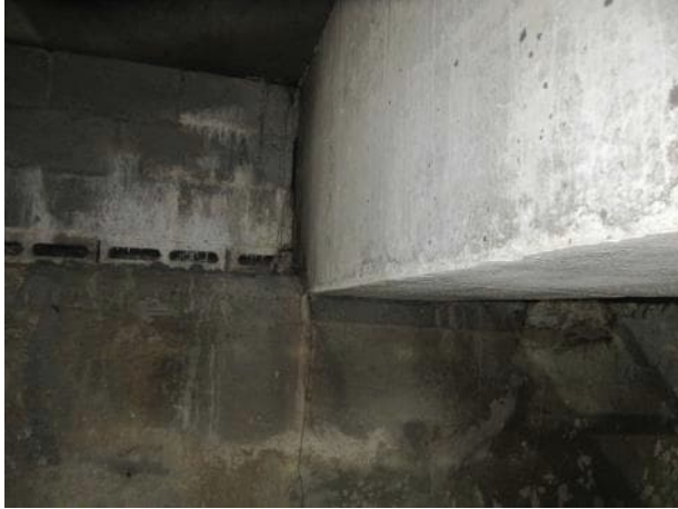
Photo 5.4.1. B16 north bearing.
