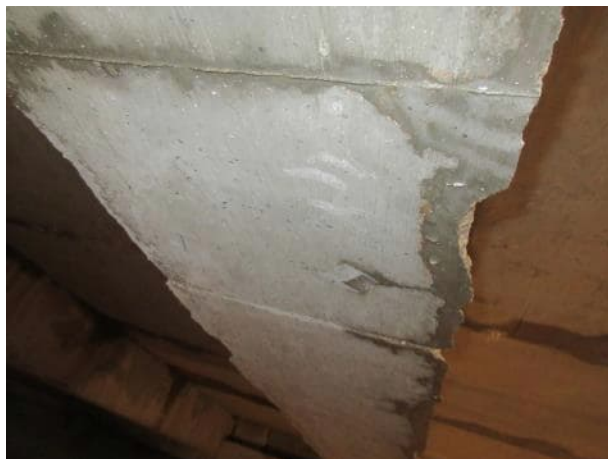
Photo 5.1.32. Underside of B5.
