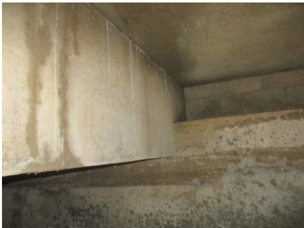
Photo 5.4.39 South bearing B18.
