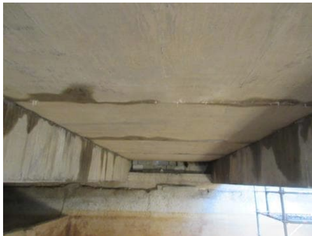
Photo 5.1.30. Underside of slabs between B4 and B5.
