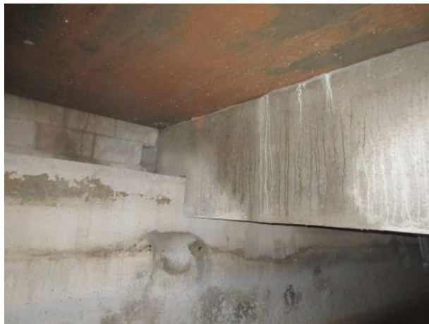
Photo 5.3.48. South bearing B14.
