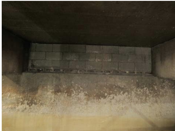
Photo 5.4.17 North bearing area between B18 and B19.
