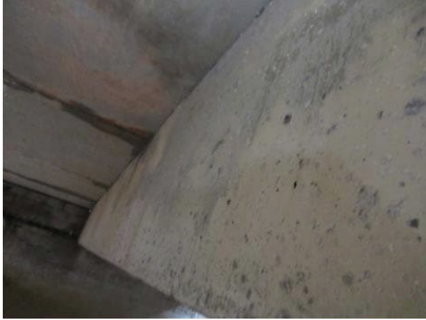
Photo 5.2.7. Beam B6 looking south.
