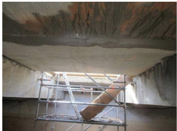
Photo 5.1.22. Underside of slab between B3 and B4.
