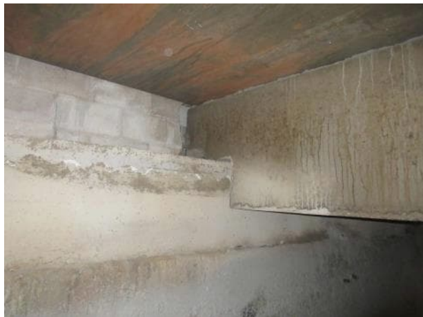
Photo 5.3.35. B12 south bearing.
