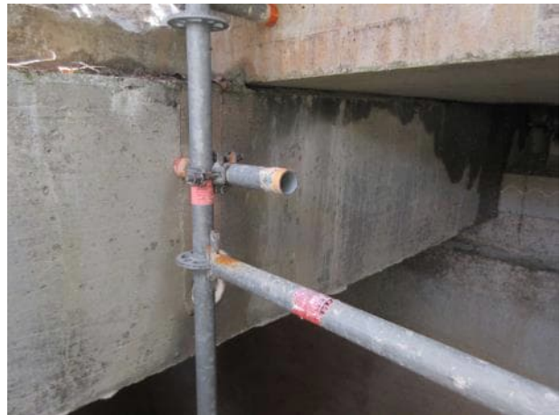
Photo 5.1.38. South end of Beam B4.
