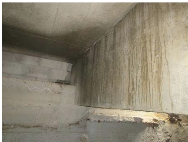
Photo 5.3.32. B11 south bearing.
