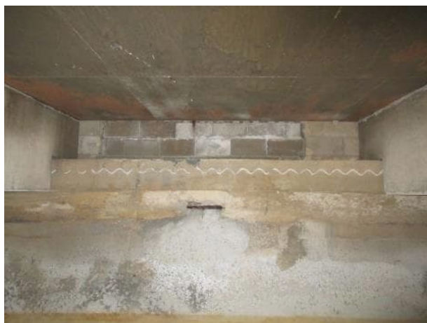
Photo 5.4.44 South bearing area between B16 and B17.
