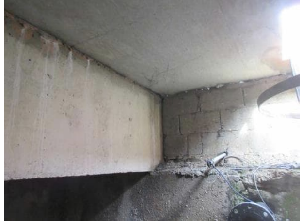
Photo 5.2.44. B7 north bearing.
