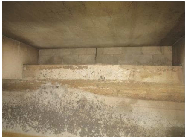
Photo 5.4.40 South bearing area between B17 and B18.
