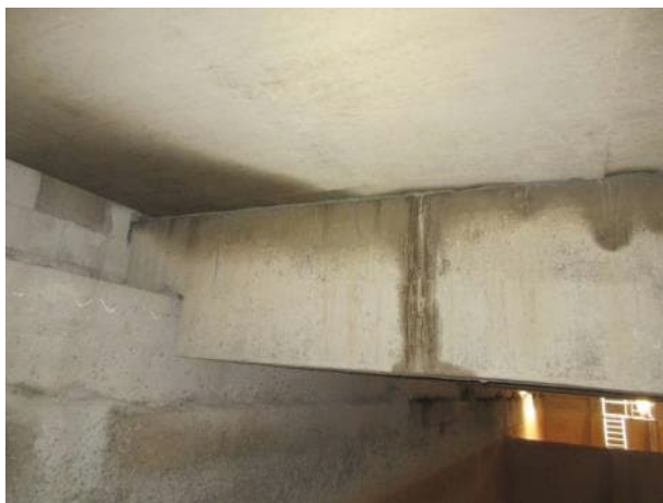
Photo 5.2.24. B9 south bearing.
