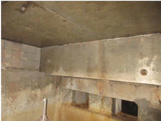
Photo 5.4.27 North bearing B20.
