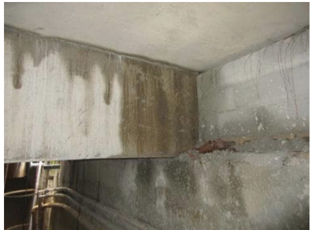
Photo 5.2.34. B9 north bearing.
