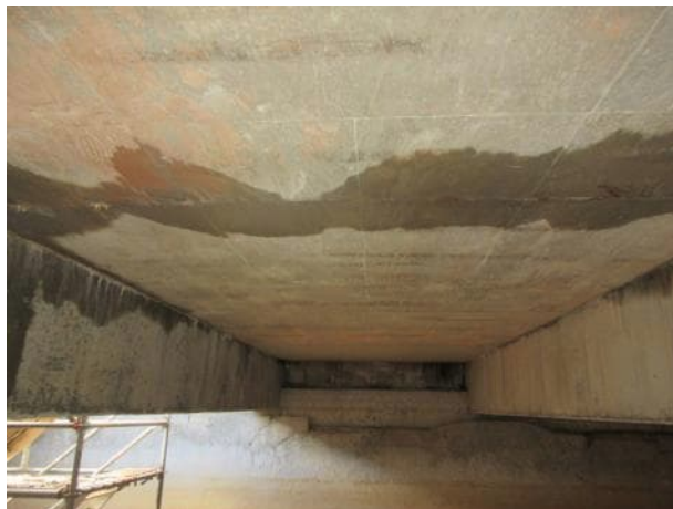
Photo 5.1.18. Underside of slabs between B2 and B3.
