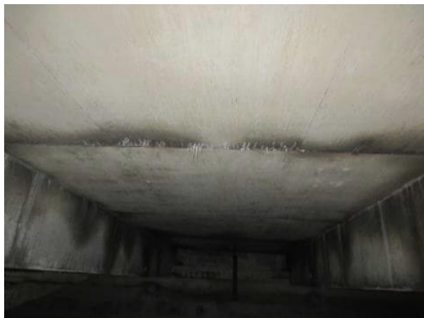
Photo 5.3.19. Slabs between B13 and B14.
