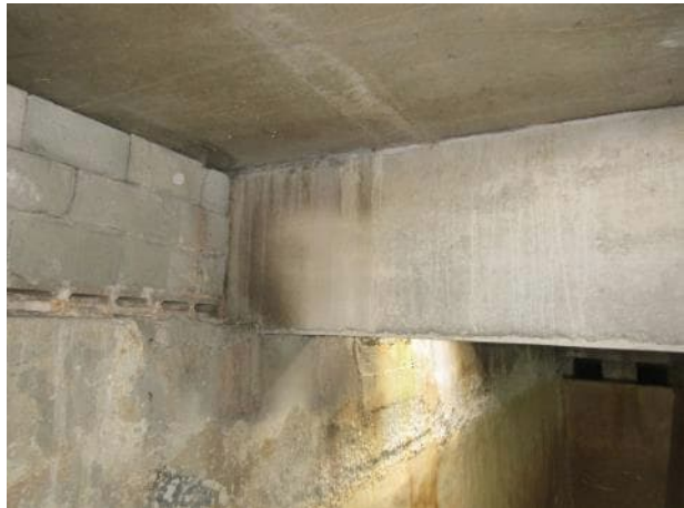
Photo 5.4.6 North bearing B17.
