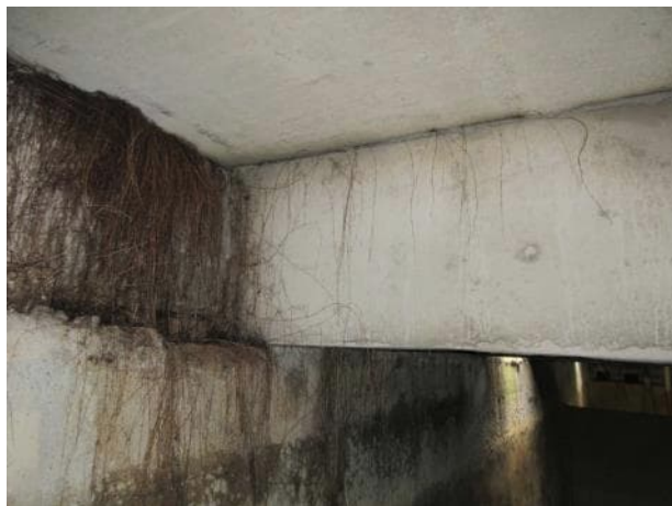
Photo 5.3.7. North bearing B12.
