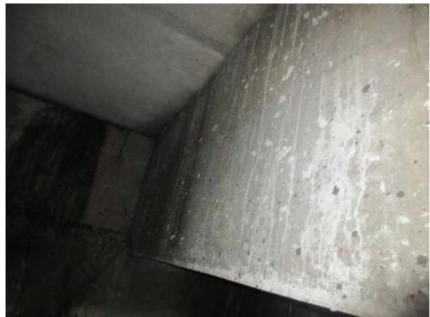
Photo 5.3.4. B11 looking north - west side.
