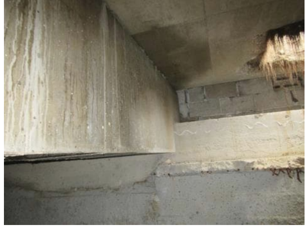
Photo 5.3.30. Beam B11 south bearing.
