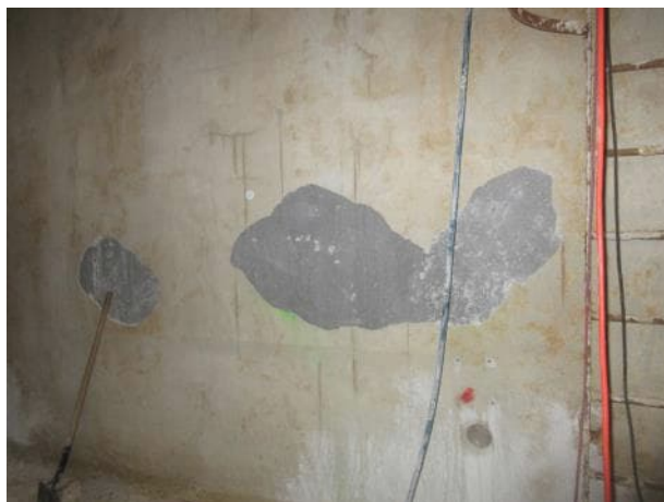
Photo 5.5.8 North wall section 2.
