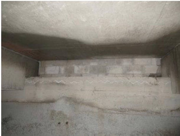
Photo 5.3.33. South bearing area between B11 and B12.
