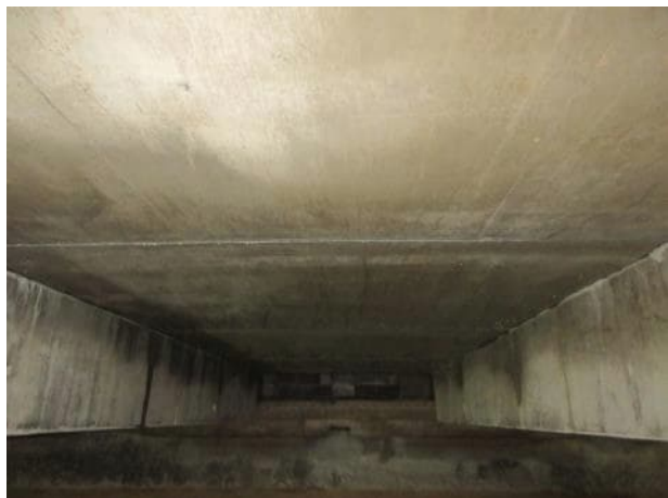
Photo 5.4.8 Underside of slabs between B16 and B17.
