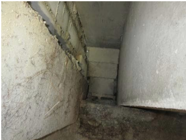
Photo 5.1.3. B1 looking north.
