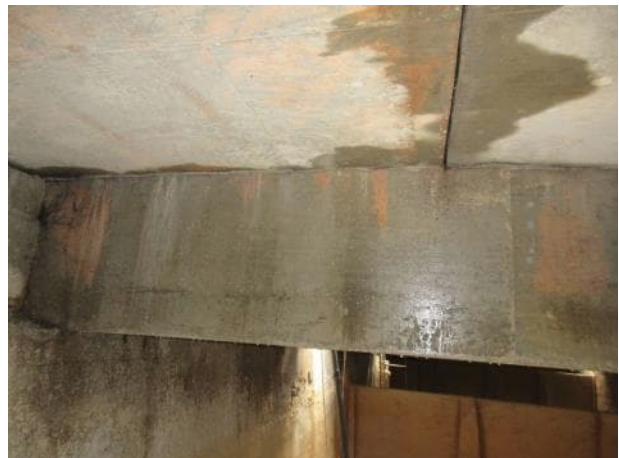
Photo 5.1.16. Beam B3 north end.
