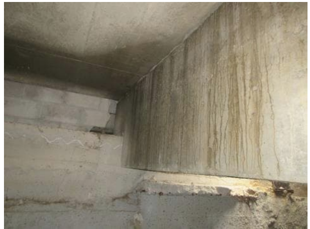
Photo 5.3.32. B11 south bearing.
