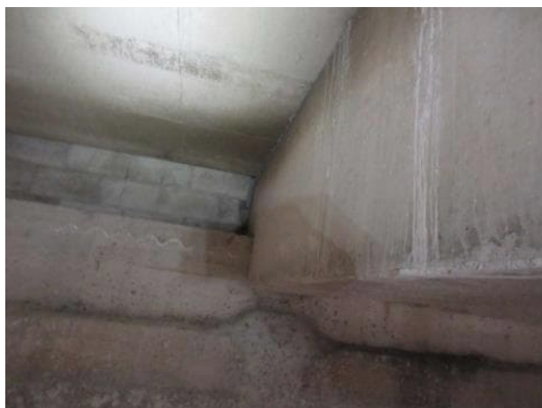
Photo 5.2.17. B8 south bearing.
