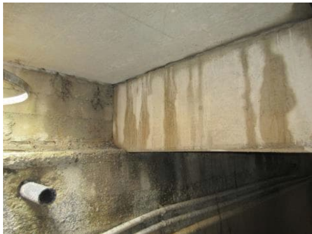
Photo 5.2.43. B8 north bearing.
