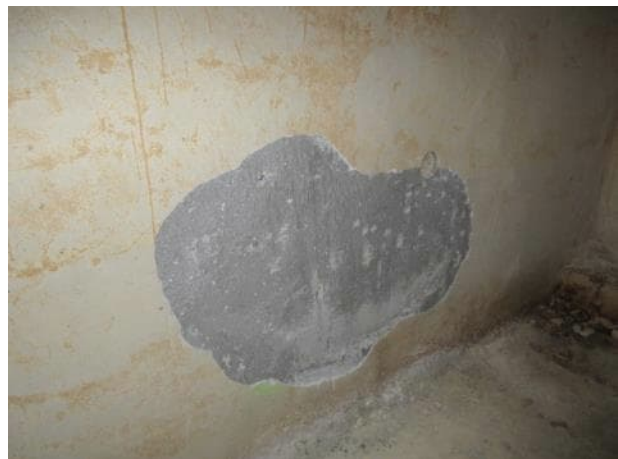
Photo 5.5.12 South wall section 2.
