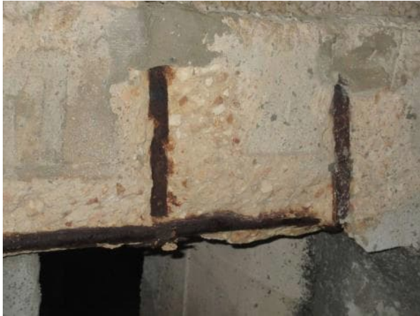
Photo 5.4.35 Corroded stirrups.
