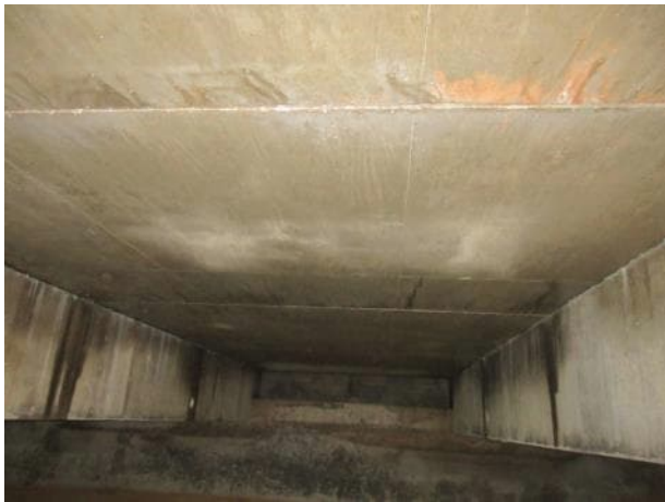
Photo 5.4.13 Underside of slabs between B17 and B18.
