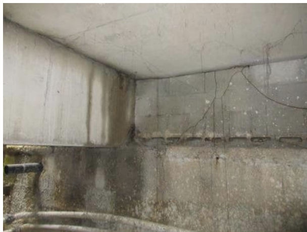
Photo 5.2.40. B8 north bearing.
