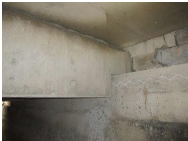
Photo 5.2.15. B8 south bearing.
