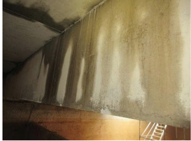
Photo 5.2.50. B5 looking south.
