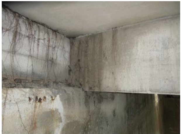
Photo 5.3.26. B15 north bearing.
