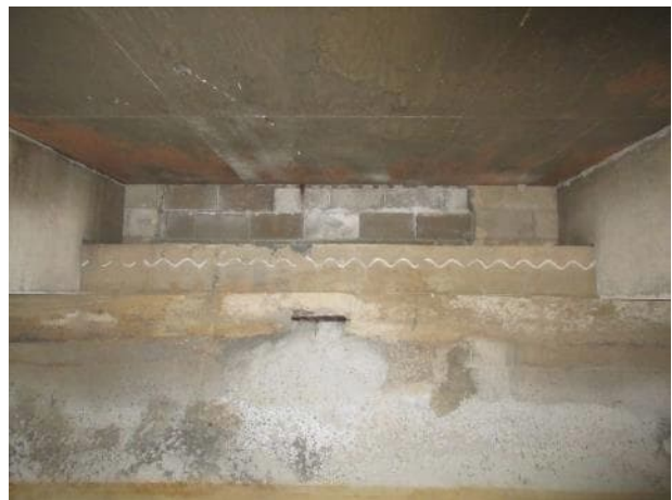
Photo 5.4.44 South bearing area between B16 and B17.
