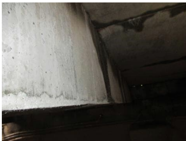
Photo 5.2.30. B10 looking north.
