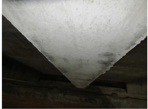
Photo 5.4.2. Underside of B16.
