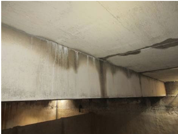
Photo 5.2.11. B7 looking north.
