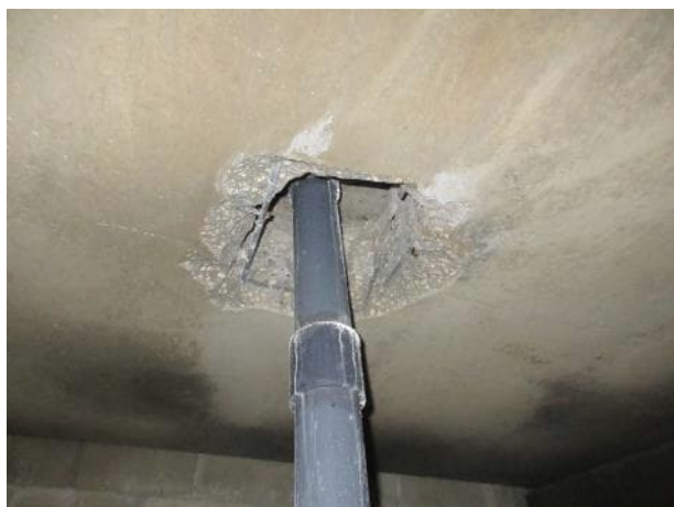
Photo 5.3.43. Opening created in the slab between B13 and B14.
