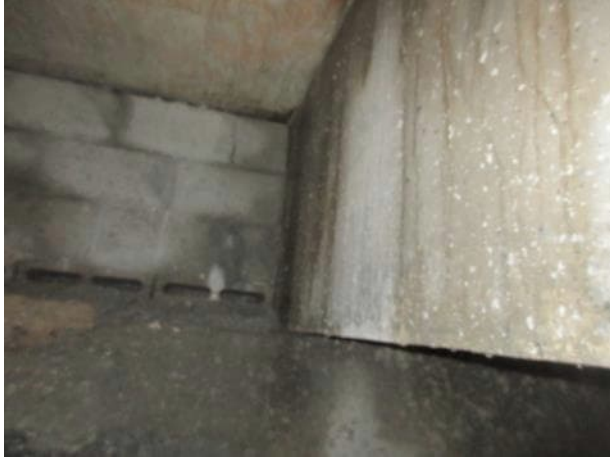
Photo 5.2.49. B5 north bearing.
