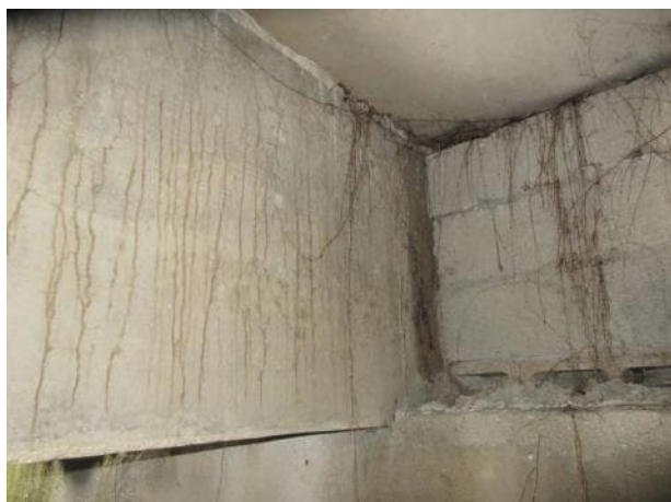
Photo 5.3.22. B14 north bearing east side.
