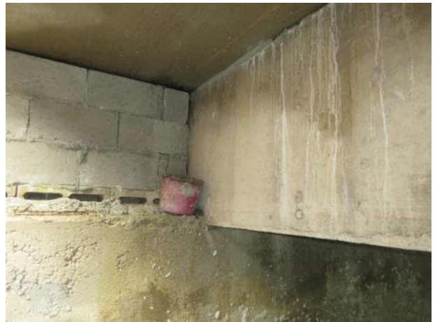
Photo 5.4.14 North bearing B18.
