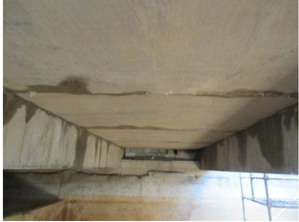
Photo 5.1.30. Underside of slabs between B4 and B5.
