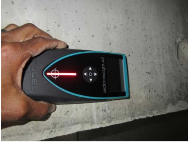
Photo 5.1.11. Rebar scan of B1.
