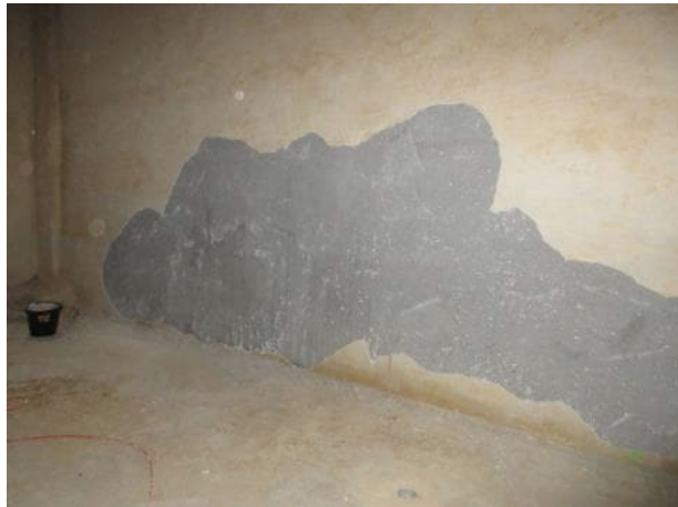
Photo 5.5.9 South wall section 2.
