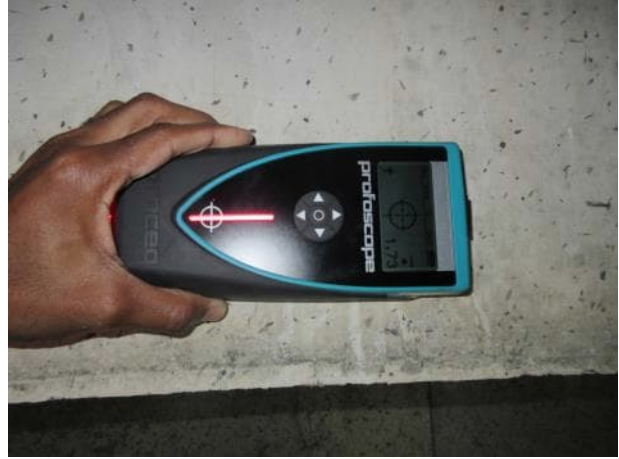
Photo 5.1.12. Rebar scan of B1.
