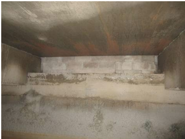
Photo 5.3.37. South bearing area between B12 and B13.
