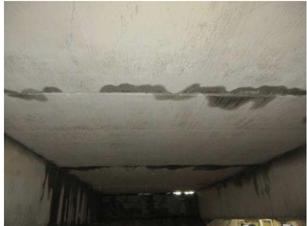
Photo 5.2.4. Underside of slab between B6 and B7.
