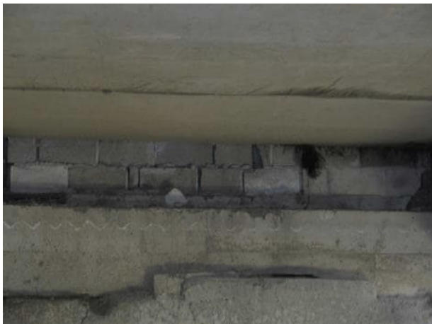
Photo 5.1.33. South bearing area between B4 and B5.
