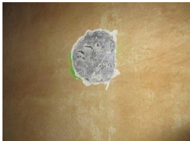
Photo 5.5.14 North wall section 1.
