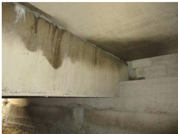
Photo 5.2.23. B9 south bearing.
