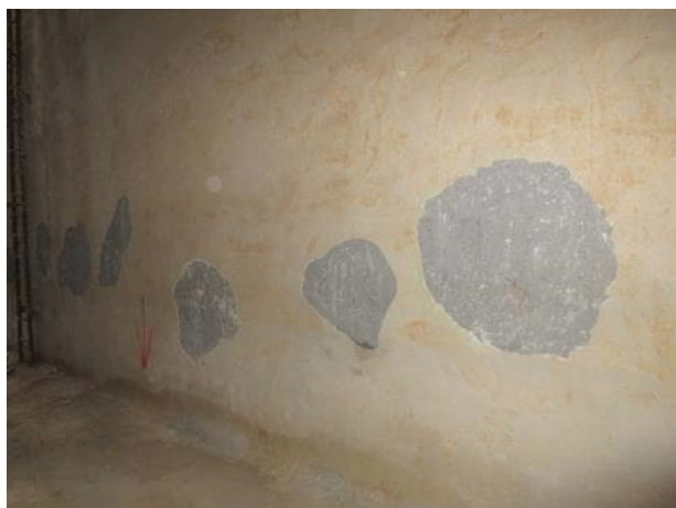
Photo 5.5.5 North wall section 2.
