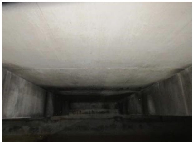
Photo 5.3.28. Slabs between B14 and B15.
