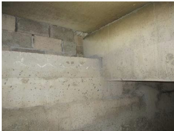
Photo 5.2.14. B7 south bearing.
