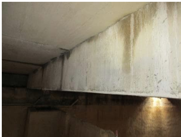
Photo 5.2.28. B10 looking north.
