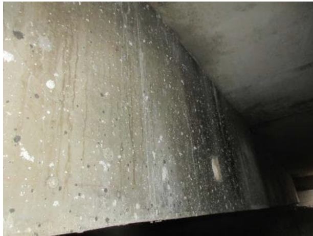
Photo 5.3.5. B11 looking west.
