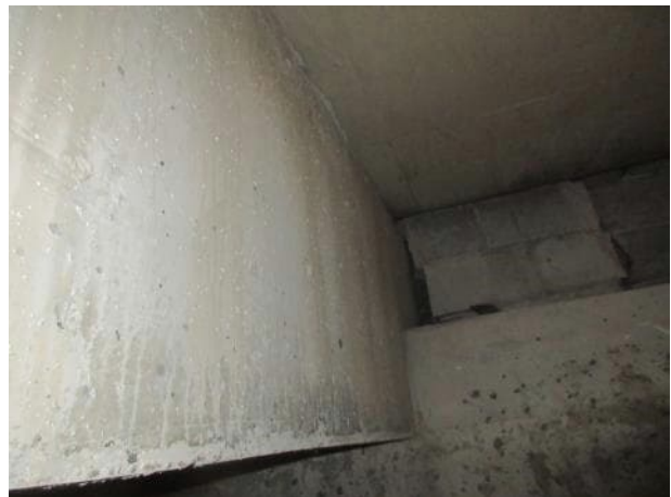
Photo 5.2.6. North Bearing B6.
