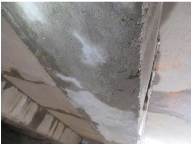
Photo 5.1.27. Old repair under B4.
