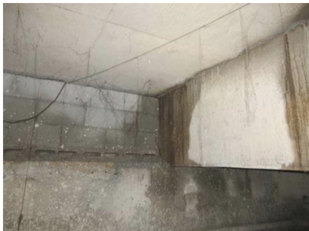
Photo 5.2.39. B9 north bearing.
