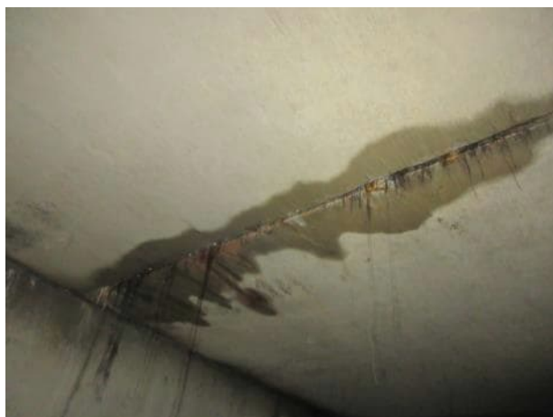
Photo 5.2.41. Root growth through slab joints between B8 and B9.
