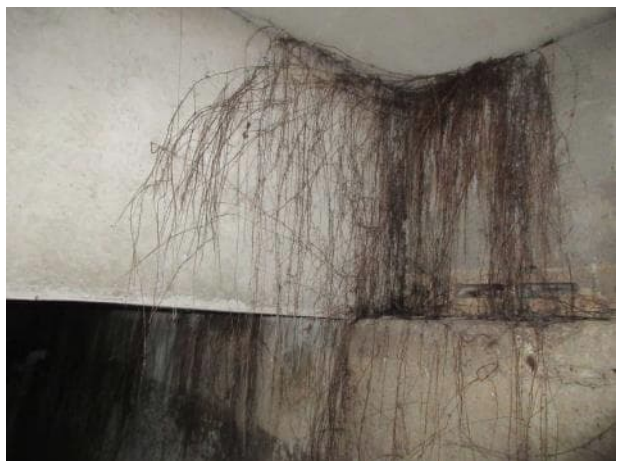
Photo 5.3.10. B12 north bearing.
