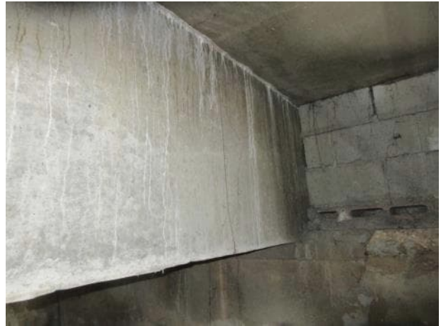
Photo 5.4.4 North bearing B16.
