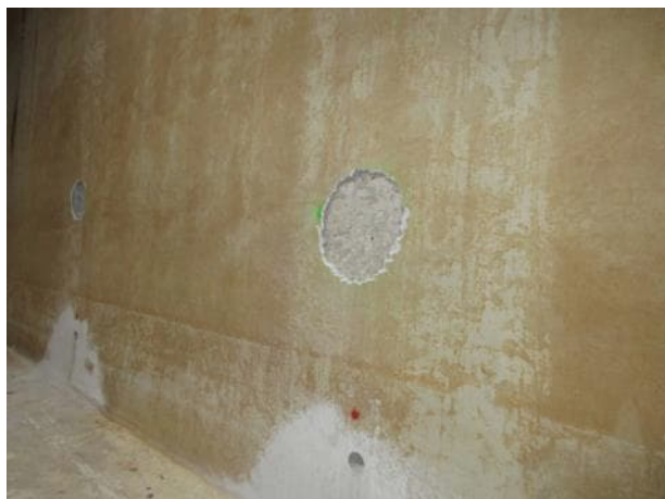
Photo 5.5.13 North wall section 1.
