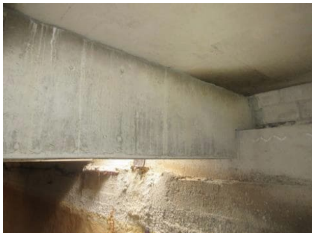
Photo 5.2.27. B10 south bearing.
