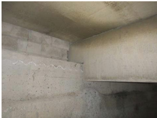
Photo 5.2.19. B8 south bearing.
