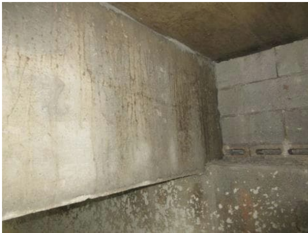
Photo 5.4.25 North bearing B19.
