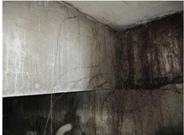
Photo 5.3.2. North bearing B11.
