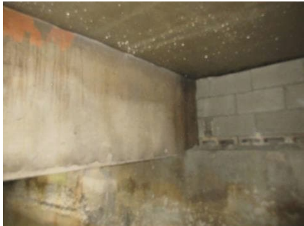
Photo 5.4.18 North bearing B18.
