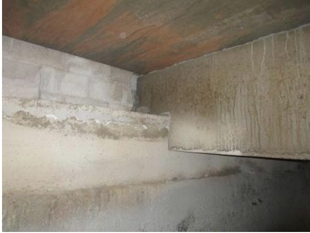
Photo 5.3.35. B12 south bearing.
