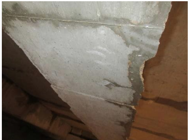
Photo 5.1.32. Underside of B5.
