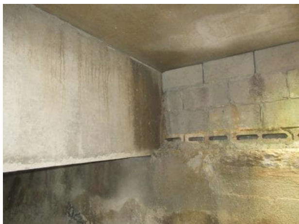
Photo 5.4.10 North bearing B17.
