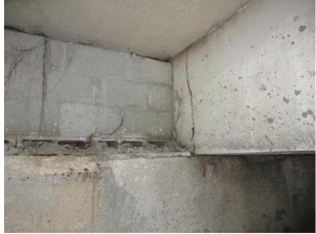
Photo 5.2.32. B10 north bearing.
