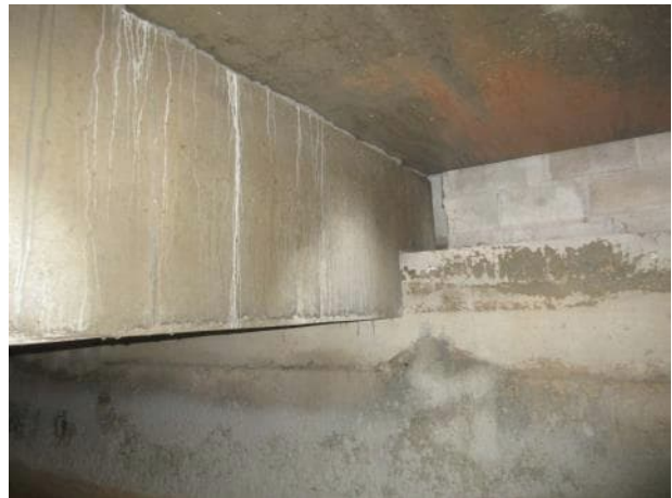
Photo 5.3.38. B13 south bearing.
