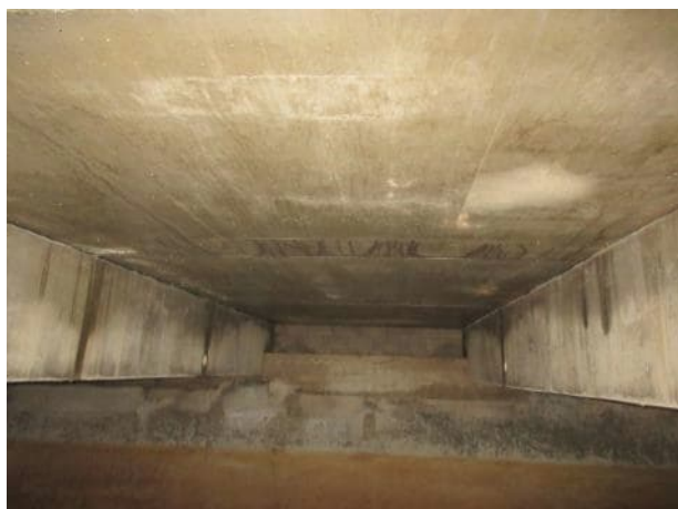
Photo 5.4.21 Underside of slabs between B18 and B19.
