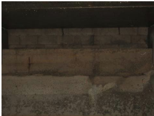
Photo 5.4.29 South bearing area between B19 and B20.
