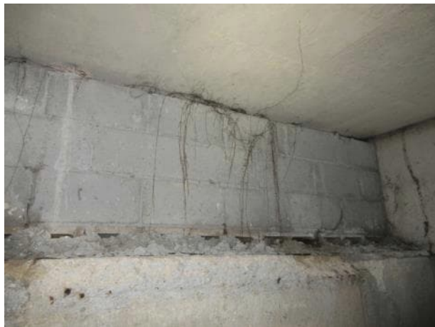
Photo 5.2.37. North bearing area between B8 and B9. Roots visible.
