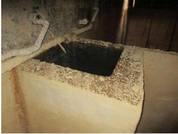
Photo 5.2.31. Water filled tower at divide wall near B10.
