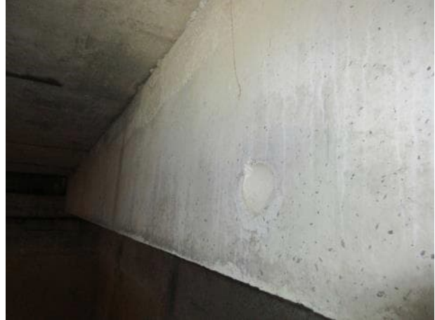
Photo 5.1.2. B1 looking south.
