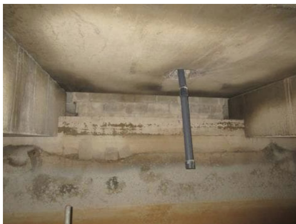
Photo 5.3.44. South bearing area between B13 and B14.
