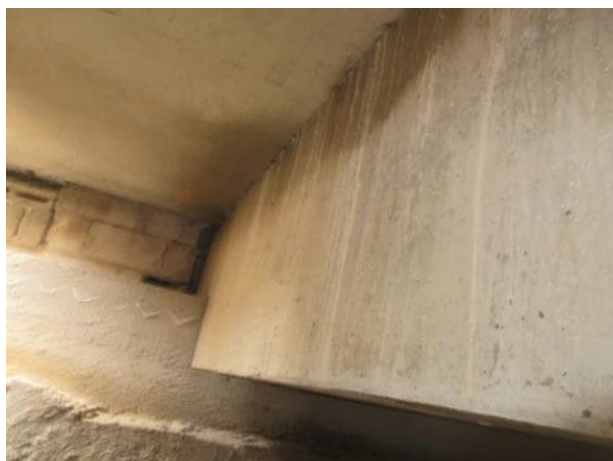
Photo 5.2.29. B10 south bearing.
