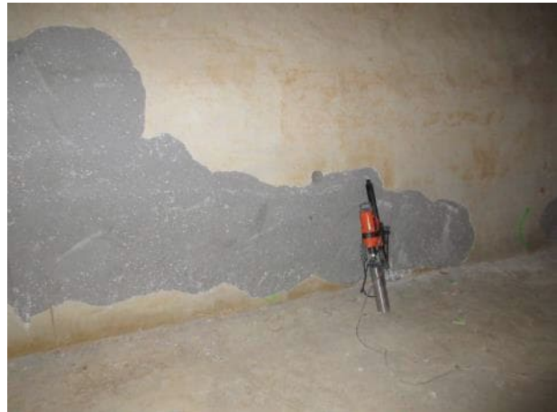
Photo 5.5.10 South wall section 2.
