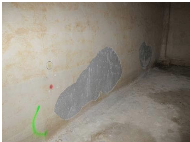
Photo 5.5.11 South wall section 2.
