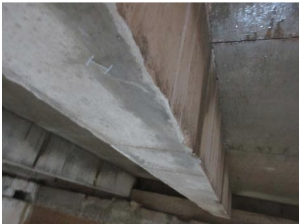
Photo 5.4.15 Underside of Beam B18.
