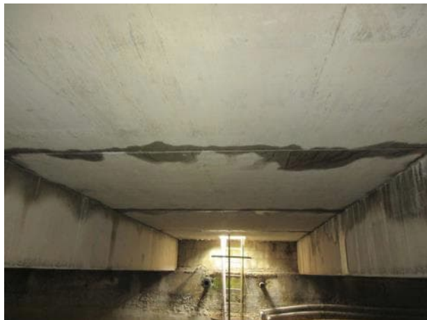
Photo 5.2.13. Underside of slab between B7 and B8.
