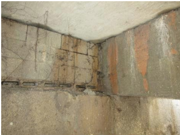
Photo 5.1.25. Beam B4 north bearing.
