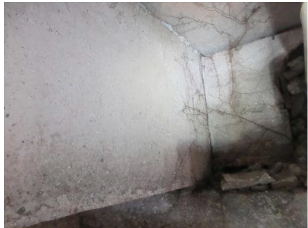
Photo 5.1.4. B1 north bearing.
