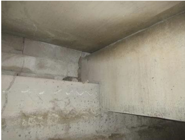
Photo 5.2.1. South end of B6 bearing.
