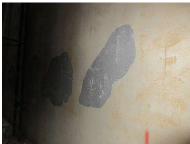
Photo 5.5.6 North wall section 2.
