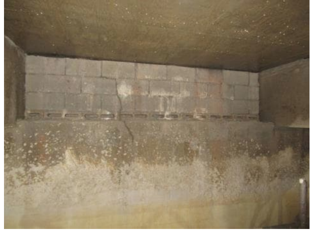
Photo 5.4.24 North bearing between B19 and B20.
