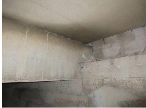
Photo 5.2.8. B7 south bearing.
