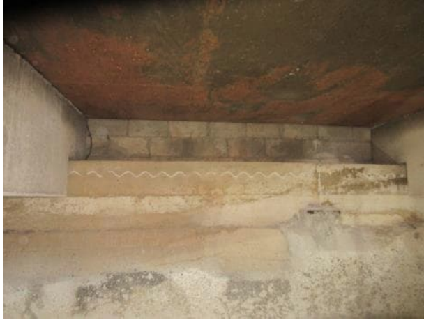
Photo 5.4.47 South bearing area between B15 and B16.
