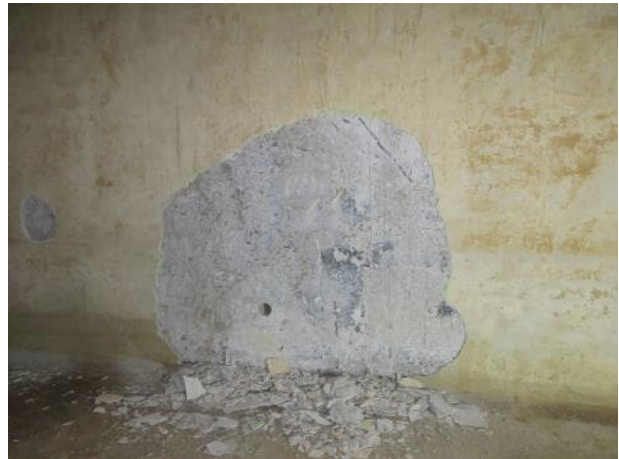
Photo 5.5.2 North wall section 3.
