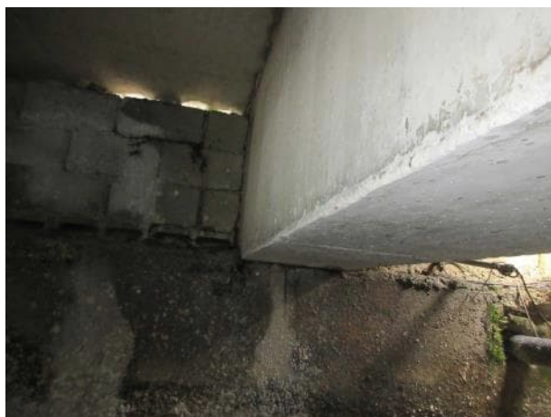
Photo 5.2.46. B6 north bearing.
