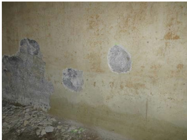
Photo 5.5.3 North wall section 3.
