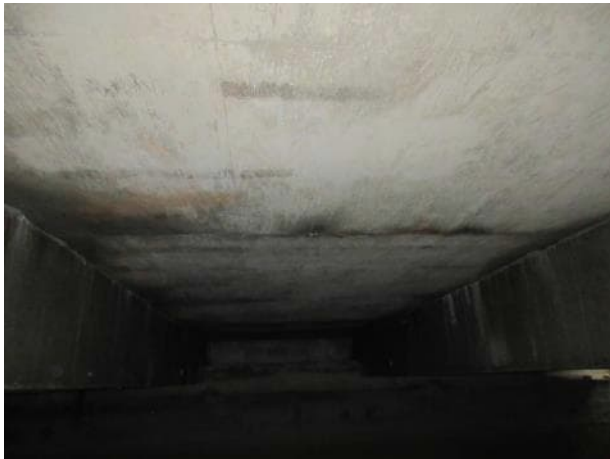
Photo 5.3.15. Slabs between B12 and B13.
