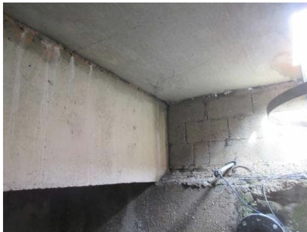
Photo 5.2.44. B7 north bearing.
