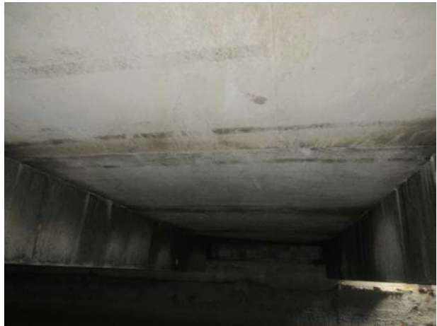
Photo 5.3.6. Slabs between B11 and B12.
