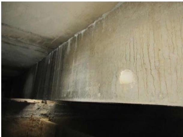
Photo 5.3.3. Beam B11 looking south.
