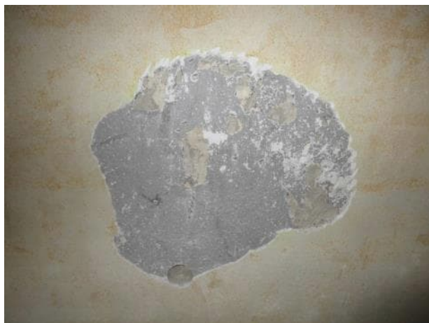
Photo 5.5.7 North wall section 2.
