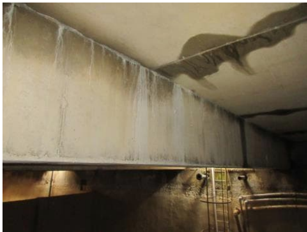
Photo 5.2.20. B8 looking north.
