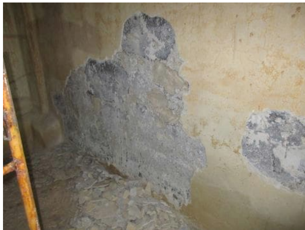
Photo 5.5.4 North wall section 3.
