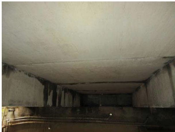
Photo 5.2.26. Underside of slab between B9 and B10.
