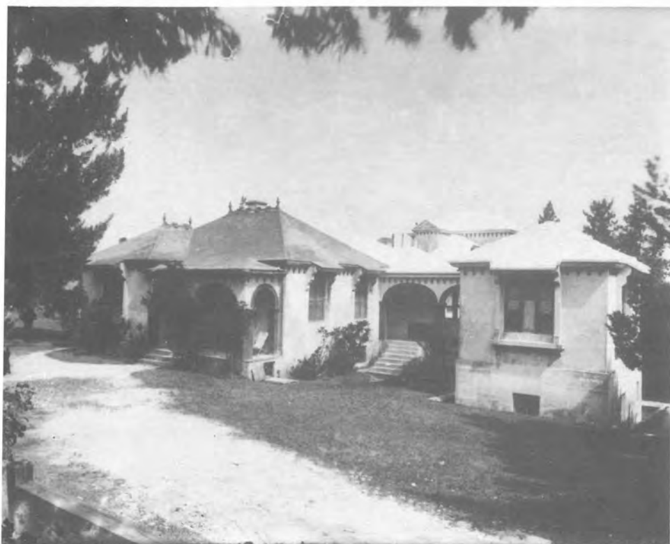
Photograph of the Cottage Hospital
